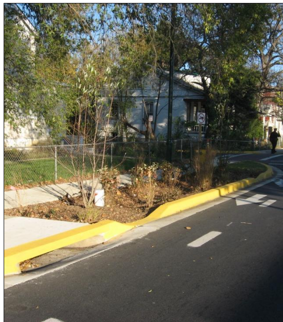
Figure 15: The retrofit of Decatur Street in Edmonston added rain gardens that capture and filter stormwater.
