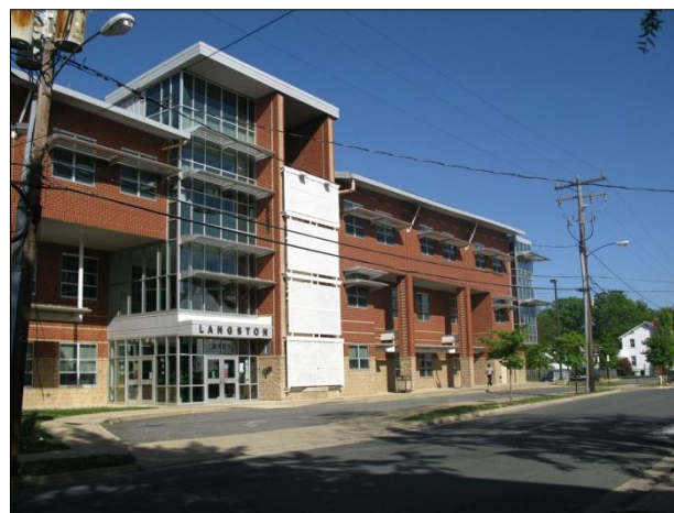
Figure 23: The Langston High School and Langston-Brown Community Center's passive survivability features include shades over windows and two 11,000-gallon cisterns, one of which is behind the white screen.
