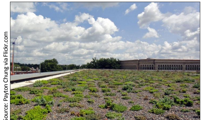
Figure 17: The Watha T. Daniel/Shaw Library in Washington, D.C., a LEED Gold building, has a roof that is part vegetated, which absorbs rainfall, and part reflective, which keeps the building cooler.
