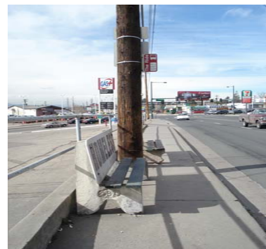
Figure 9: Narrow sidewalks along Leetsdale Drive result in signs, bus stops or utility poles in the middle of the sidewalk. (Photo courtesy of EPA)
