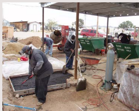
Courtesy of Tohono O'Odham Community College: Project on Carbon-Negative Building Materials
