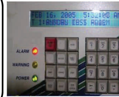
ATG in alarm status
