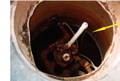
Sensor has been moved and cannot detect liquid
