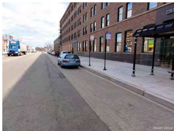
Figure 60: Permeable pavers mark a bike lane and parking area. The pavers contain a special compound to absorb nitrogen oxides.
