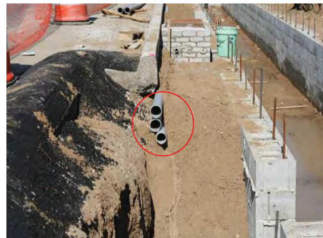
Figure 55: Construction photo showing utility conduits.
