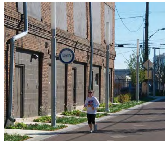
Figure 66: Downspouts flow into stormwater basins along the Trail.
