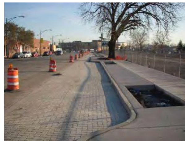
Figure 61: Cermak Road after construction of permeable parking/bike lane, stormwater storage, and sidewalk planters.
