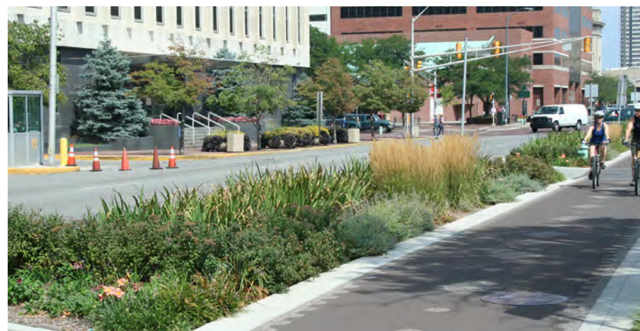
Figure 5: Raingardens along the Indianapolis Cultural Trail collect and absorb stormwater runoff. These gardens are an example of green infrastructure. Image provided by the City of Indianapolis.
