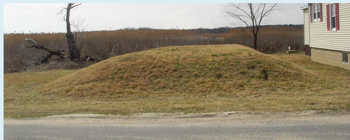
As sea level rises, the water table rises as well, which can prevent ordinary septic systems from working properly. The owner of this house in Pickering Beach responded by shifting to a mounds-based system, which provides the required separation between the drain field and the water table. © James G. Titus; used by permission.
