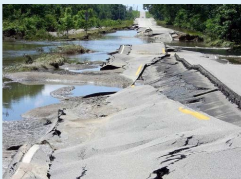
Flooding of the Cedar River in 2008 damaged this section of U.S. Highway 6 east of Atalissa. Credit: Iowa Department of Transportation.
