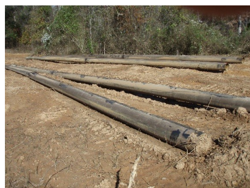
Asbestos Coated Pipeline
