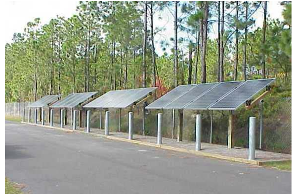
Figure C-2. Photovoltaic Solar Panel Installation.
