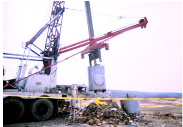
Figure C-10. LFG Well Drilling.
