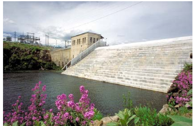
Figure C-11. 3 MW Small Hydro Plant.
