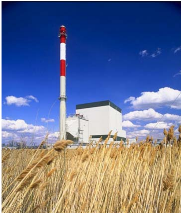
Figure C-7. 35 MW Biomass Combustion Plant.
