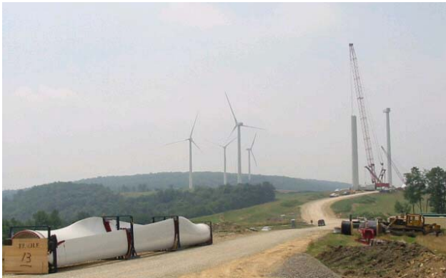
Figure 5-11. Mill Run Under Construction. (source: www.newwindenergy.com )
