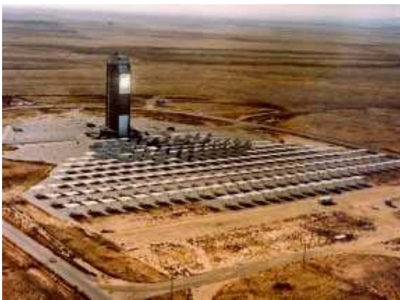
Figure C-3. Central Receiver Installation
