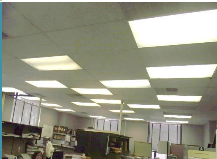
Figure 8. Significant Overlighting
