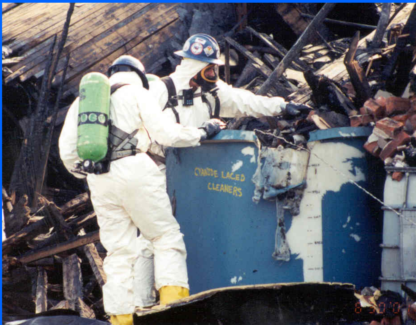
Chemical Plating Facility Fire – Detroit, MI - 2001
