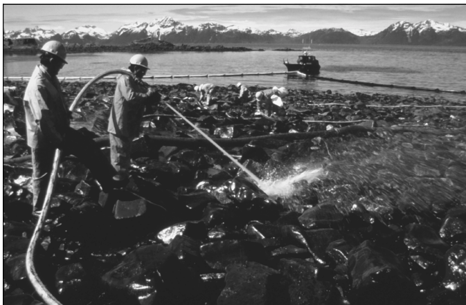
Response crews using high pressure hose to wash an oil covered beach.
