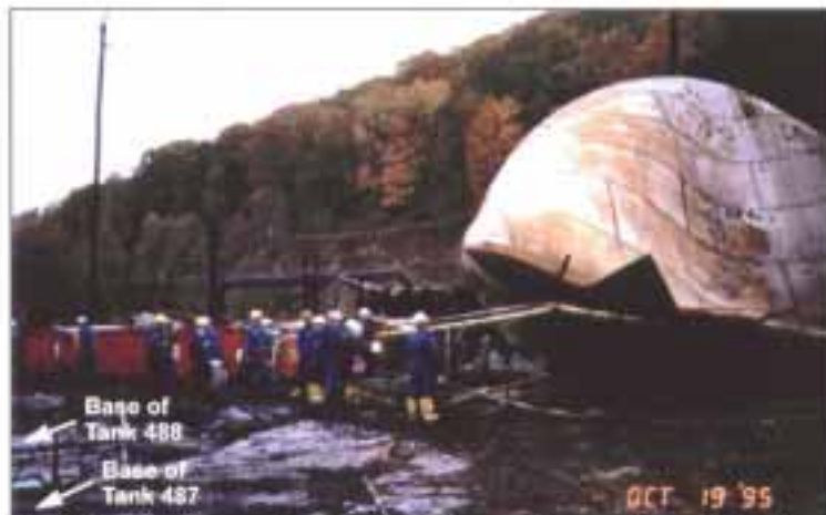
B. Dips in ground showing the original site of tanks 487 & 488. Tank 487 in background.
