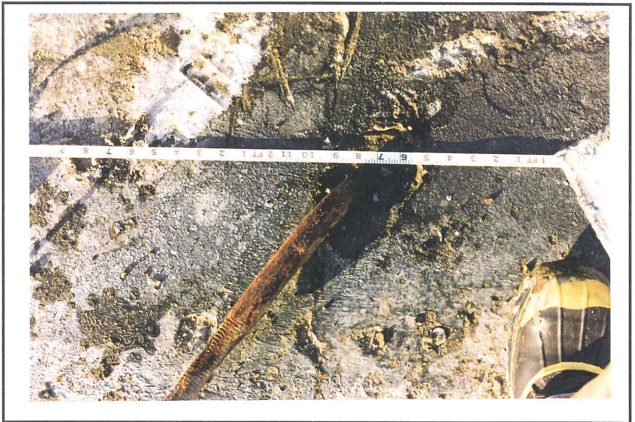
Photo 8 - 10 AN Scrubber Mounting Bolts
