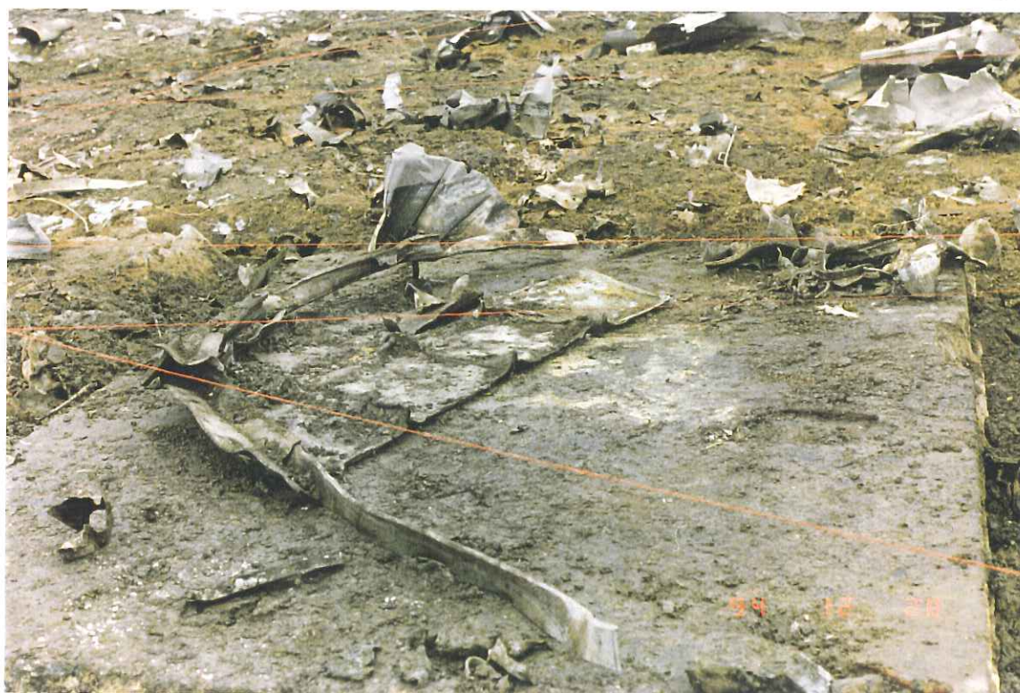
Photo 8 - 3 AN Scrubber Pad and Vessel Floor
