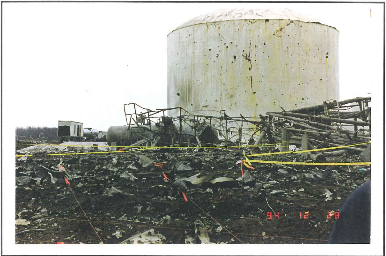
Photo 8 - 12 Water Tank Damage (Ammonia Tank Background)
