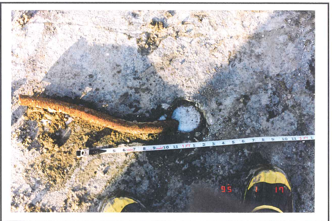
Photo 8 - 11 AN Scrubber Mounting Bolts
