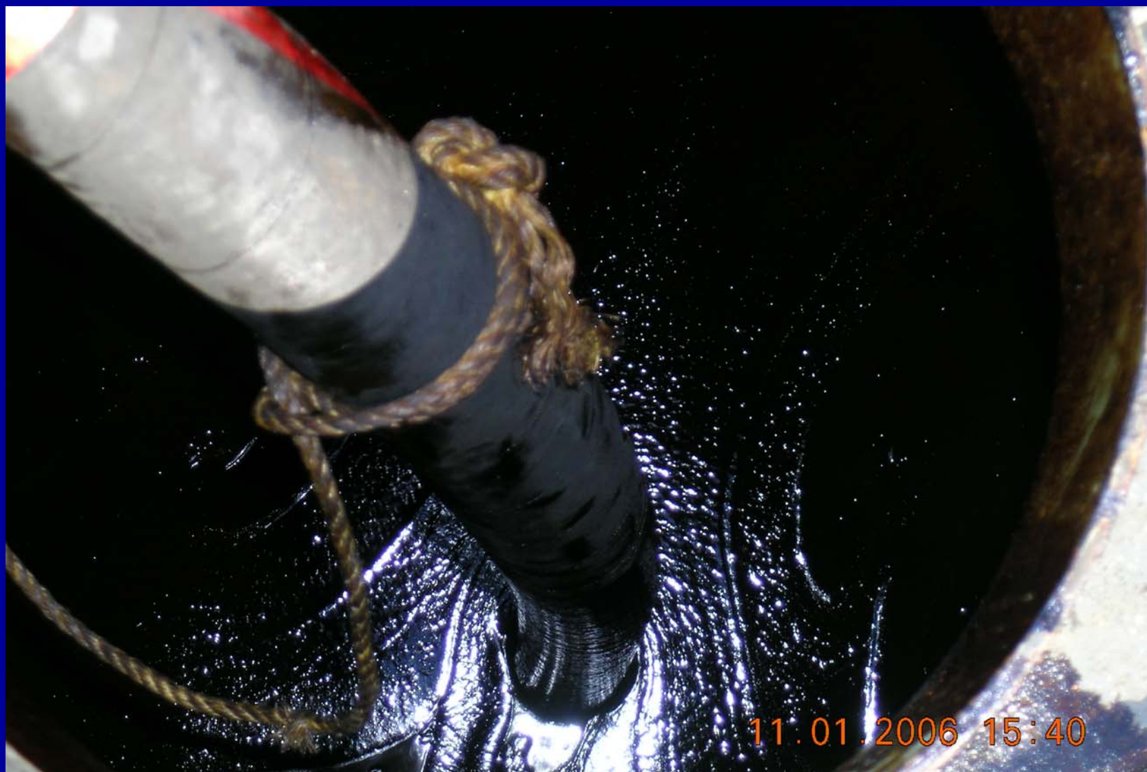
This photo shows heavy concentrations of oil remaining in one of the storage tanks (after water decanting operations had taken place).
