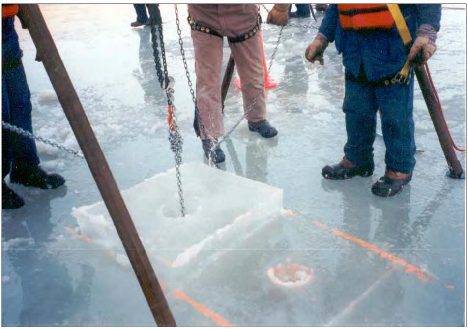
STEP 8. - LIFTING of 1st ICE BLOCK with "A" FRAME & HOIST & PUSHING ICE to SIDE
