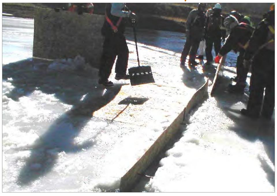
PLYWOOD SHEET BEING PLACED in "J" PORTION of THRU ICE BARRIER
