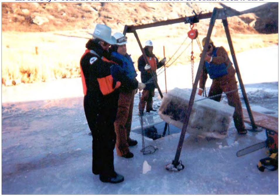
STEP 9. - LIFTING of 2nd ICE BLOCK with "A" FRAME & HOIST & "T" BAR
