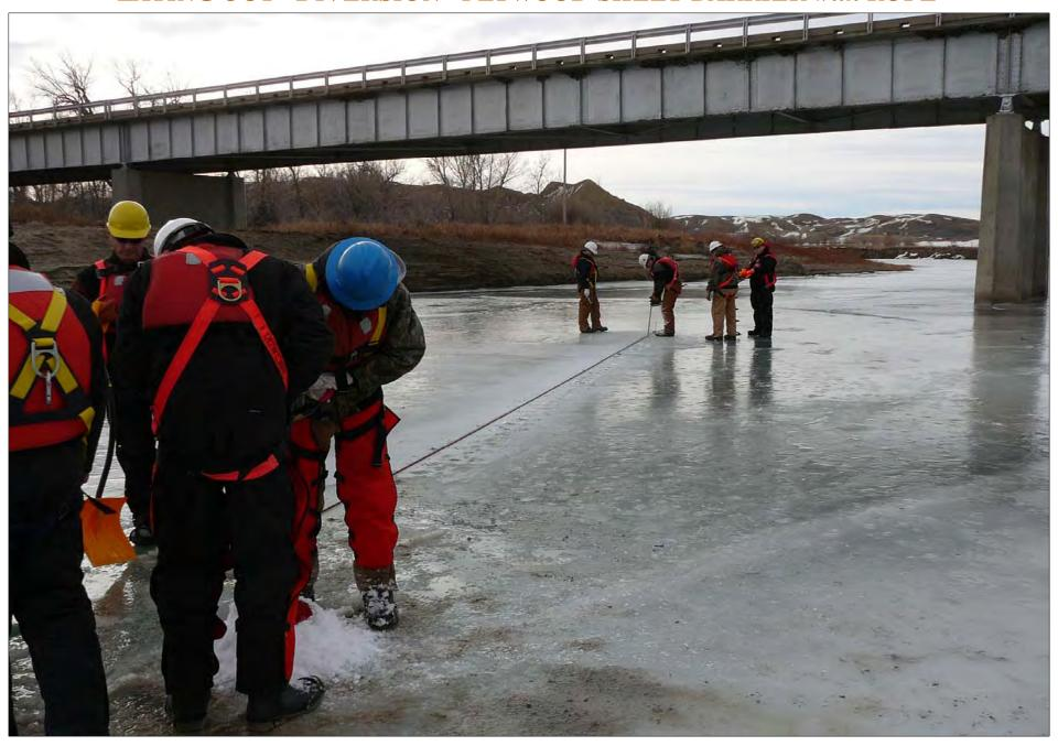
ETCHING BARRIER PATTERN with CHAIN SAW
