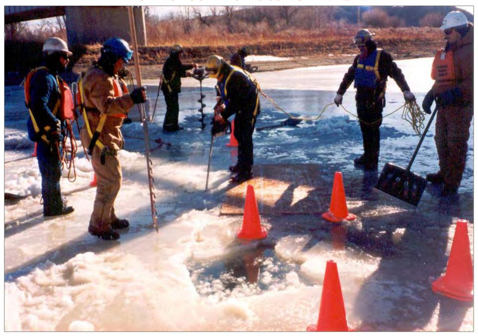
1st PLYWOOD SHEET with SPIKES to STABILIZE it on ICE
