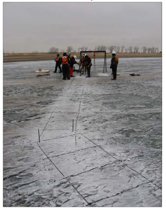
STEP 4. ICE SLOT OUTLINED with SQUARE PATTERN & AUGER HOLES DRILLED
