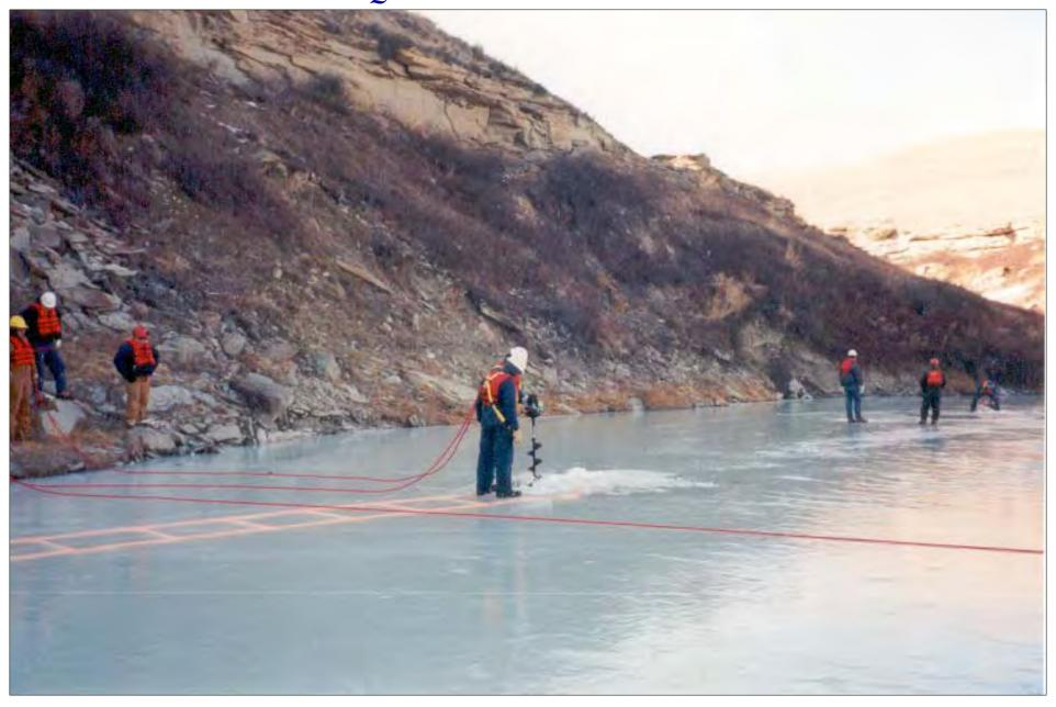
STEP 5. - CONSTANT CLEANING of ICE & SNOW from ICE SLOT DESIGNS
