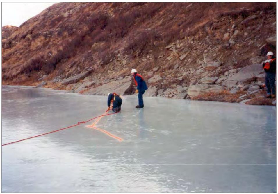
STEP 3. -LAYOUT ICE SLOT DESIGN by CHAIN SAW ETCHING
