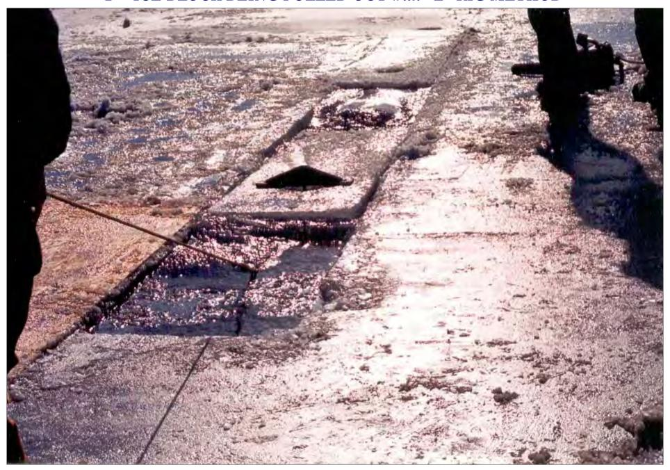
4" x 4" x 6' USED as ANCHOR POST for "Z" RIG to HAUL 8' to 10' ICE BLOCK from ICE SLOT
