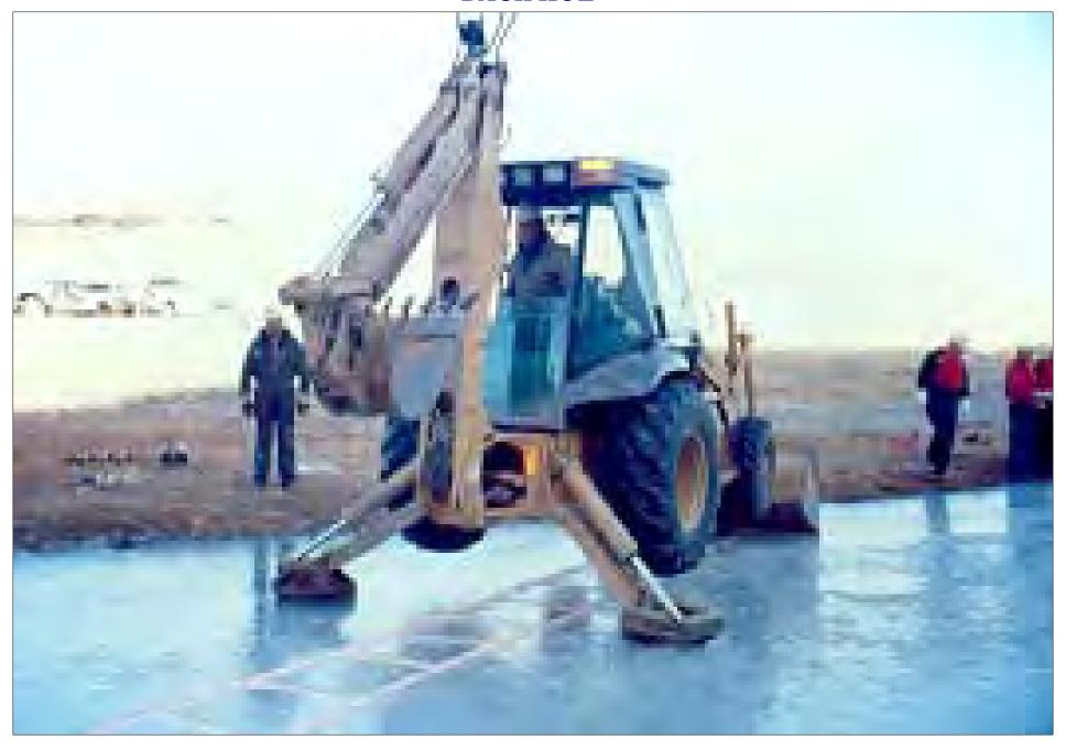
STEP 1. - INSPECT ICE for CRACKS & DETERMINE ICE SLOT POSITION
