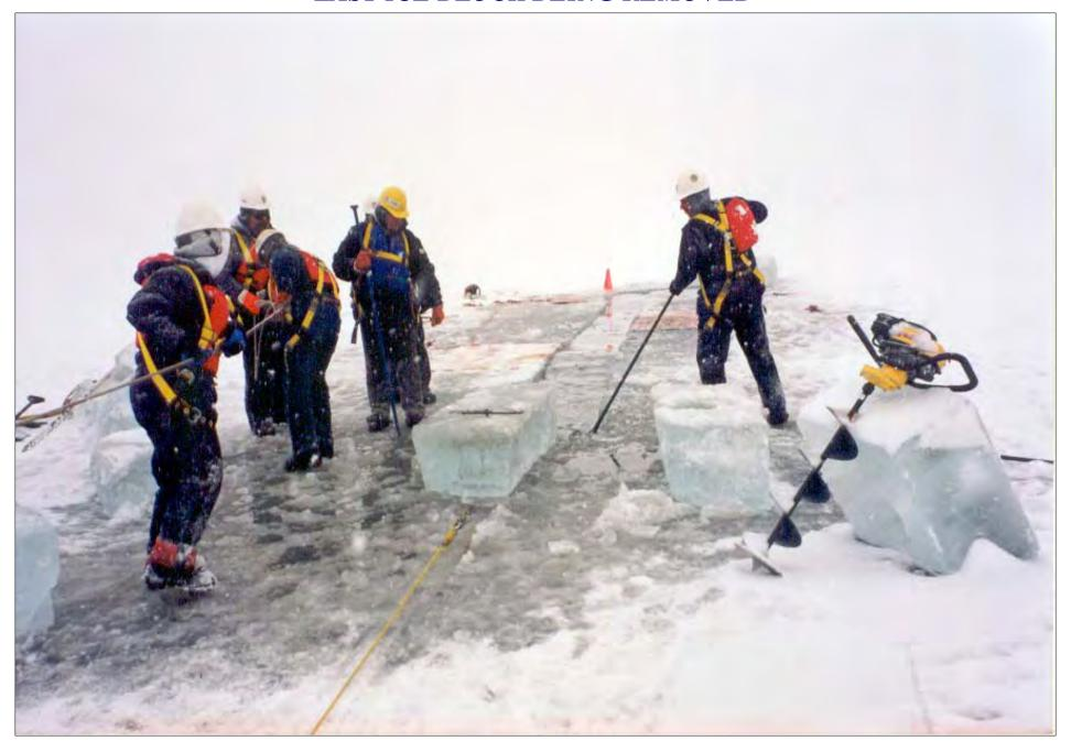
8 to 10' ICE BLOCK BEING HAULED OUT with "Z" RIG
