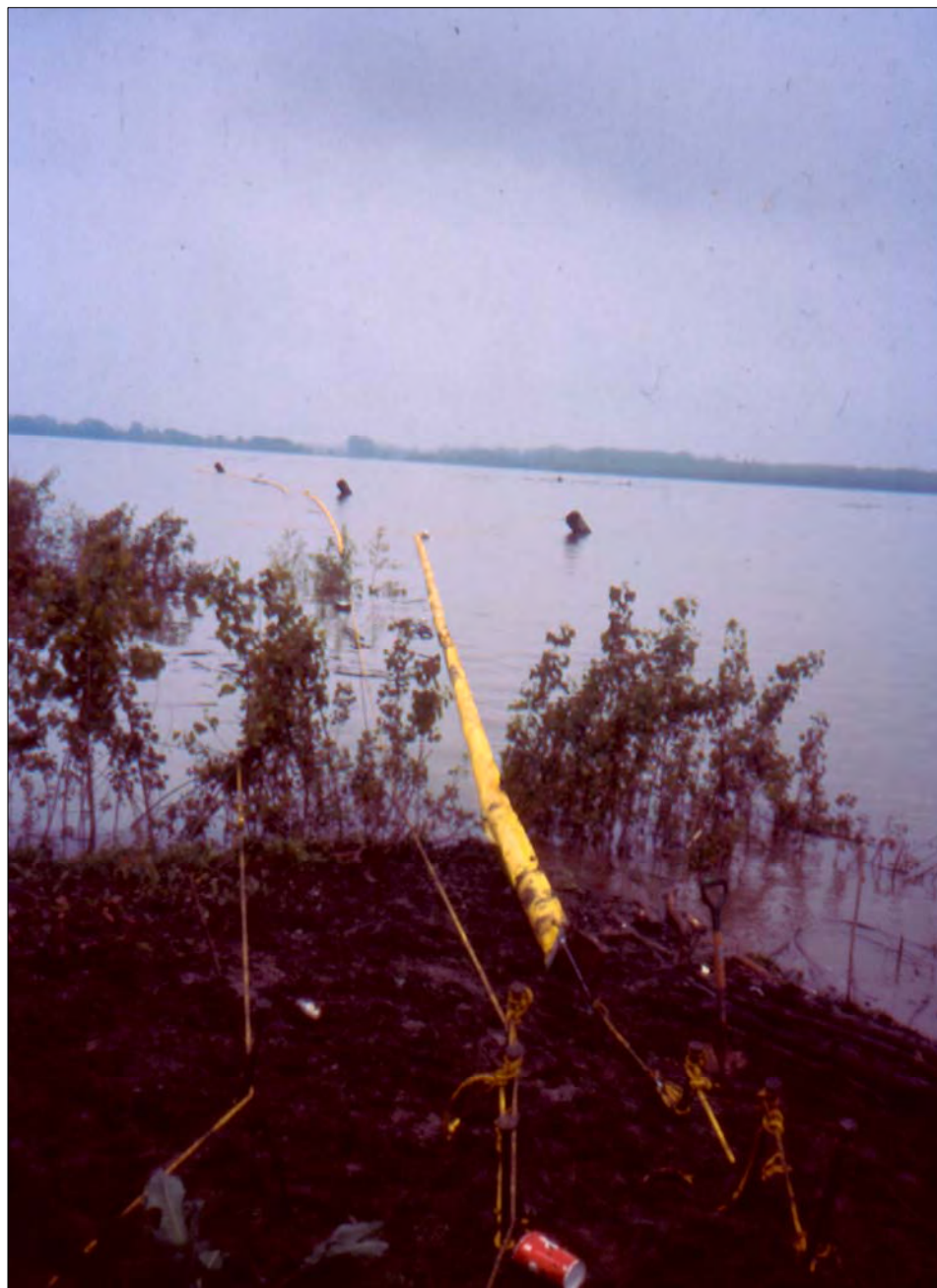
Buoy to Bank Rope Anchor System Mississippi River - St. Louis, Missouri Area
