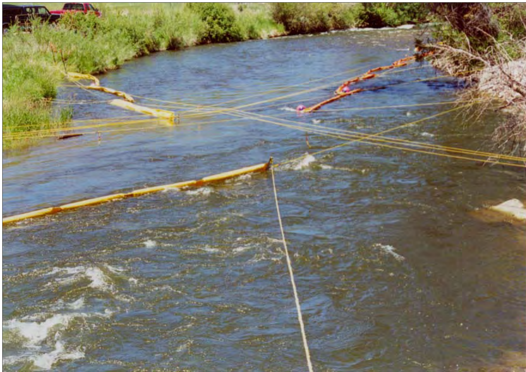
Deflection Booming - River Deployment Weber River - Coalville, Utah Area
