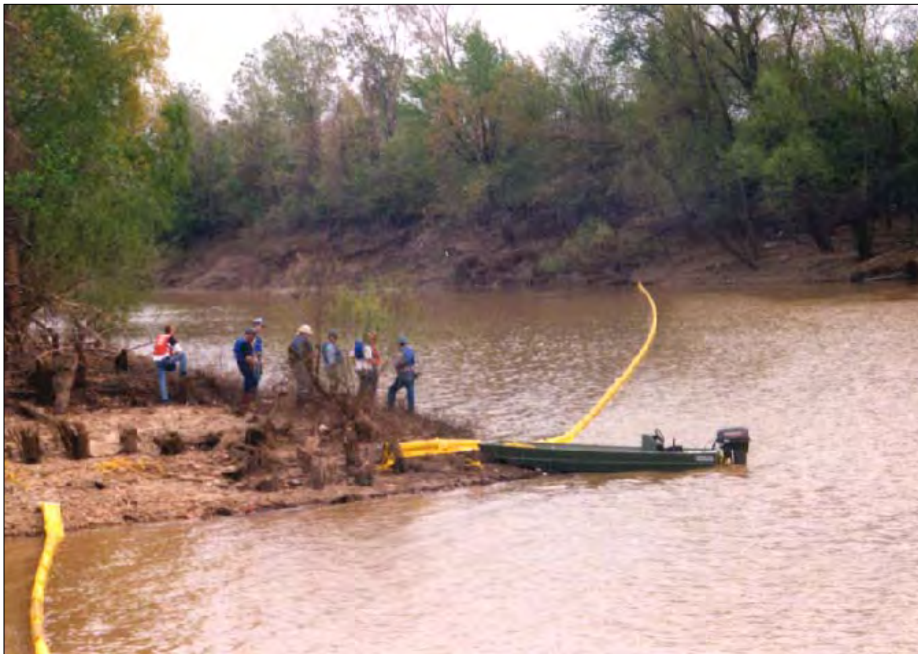
Exclusion Booming of Confluence of Rivers Nonconnah Creek - Memphis, Tennessee Area
