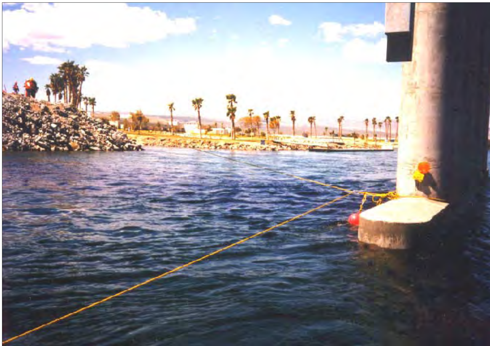
Bridge to Bank Rope Anchor System Rope Lead Anchor Collar Around Bridge Column Colorado River - Bullhead City, Arizona Area
