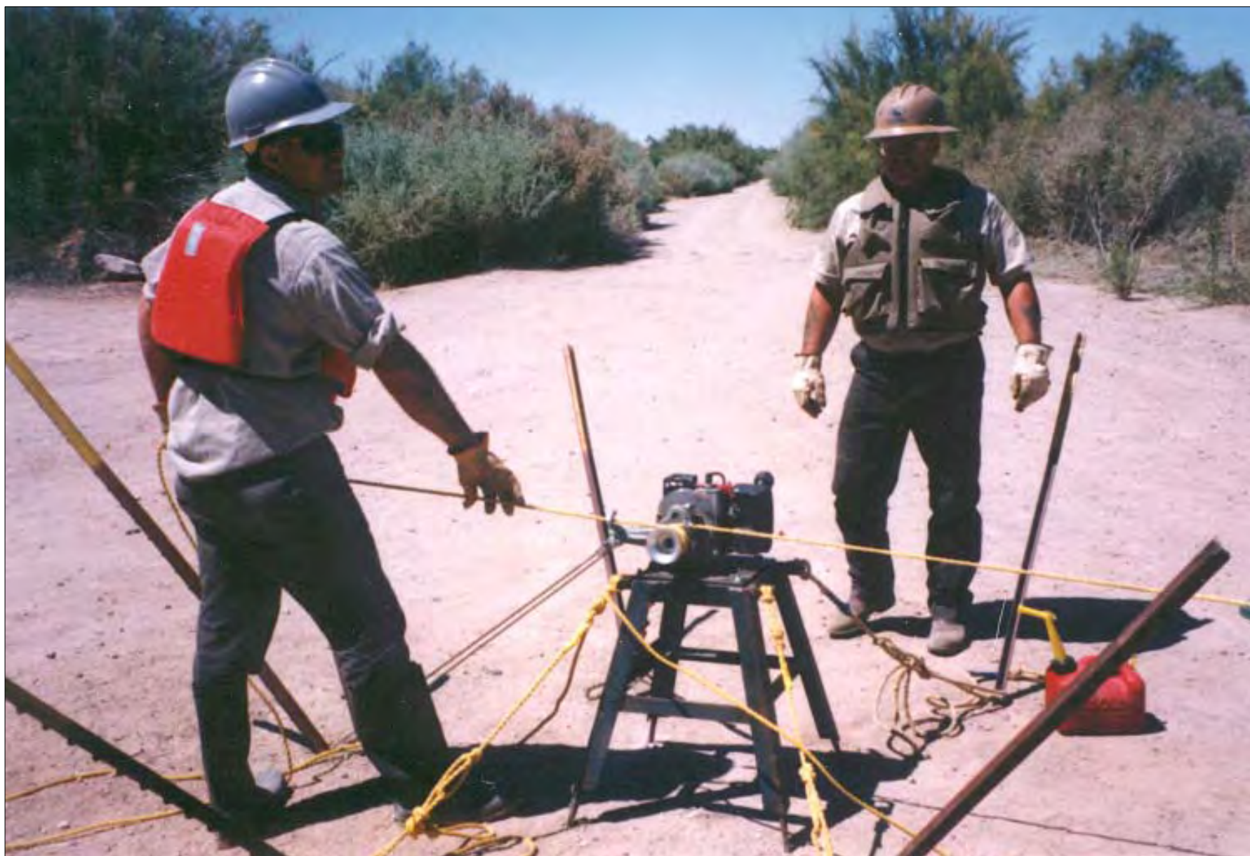
Bridge to Bank Rope Anchor System Power Wench with Rope Lead thru “D” Ring located on Bridge Column Colorado River - Blythe, California Area
