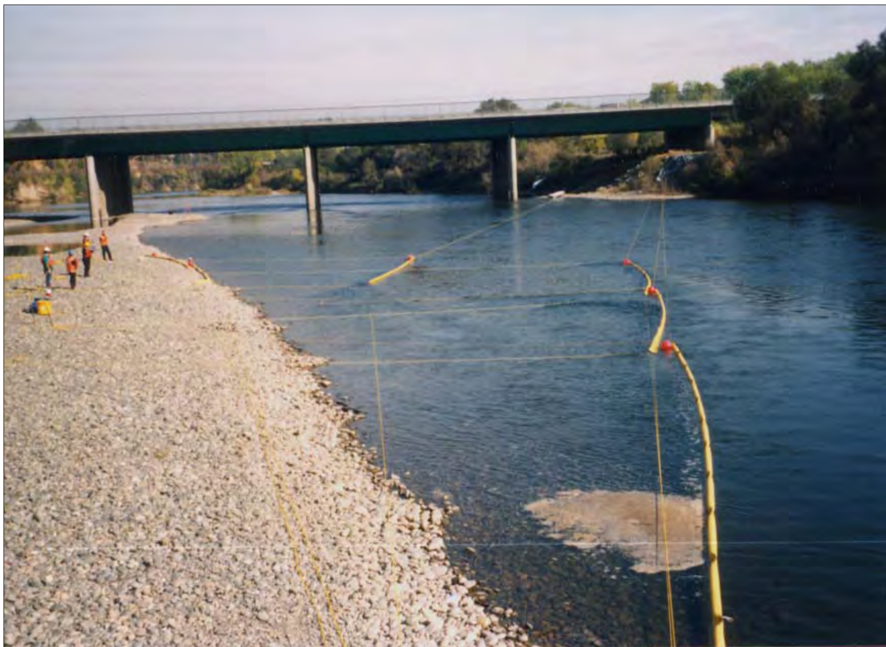
No. 4 - Boom Being Deployed - Bank to Bank Rope Anchor System American River - Sacramento, California
