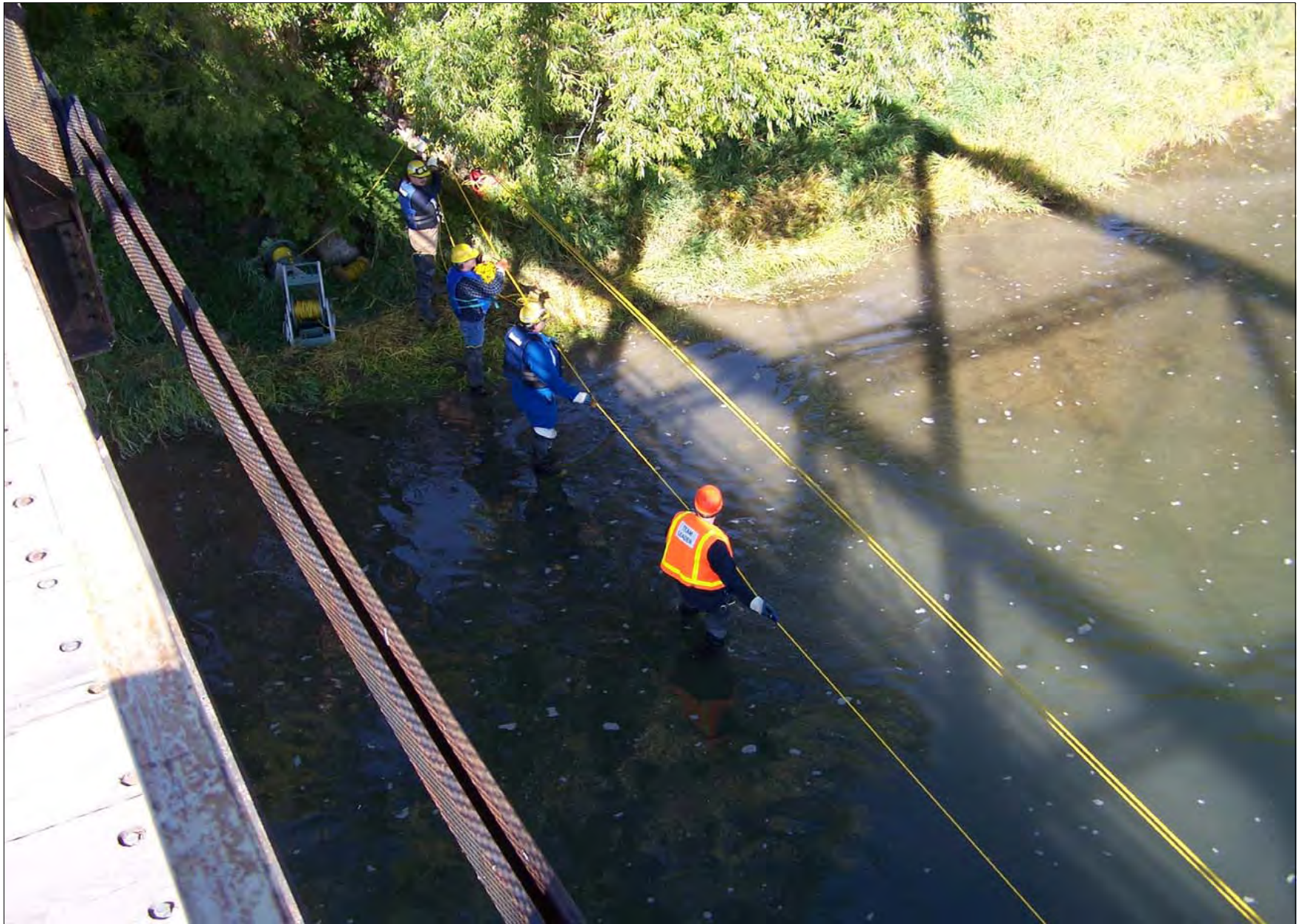
Bridge to Bank Rope Anchor System - Bridge Column to Bank Anchor Missouri River - Fort Benton, Montana
