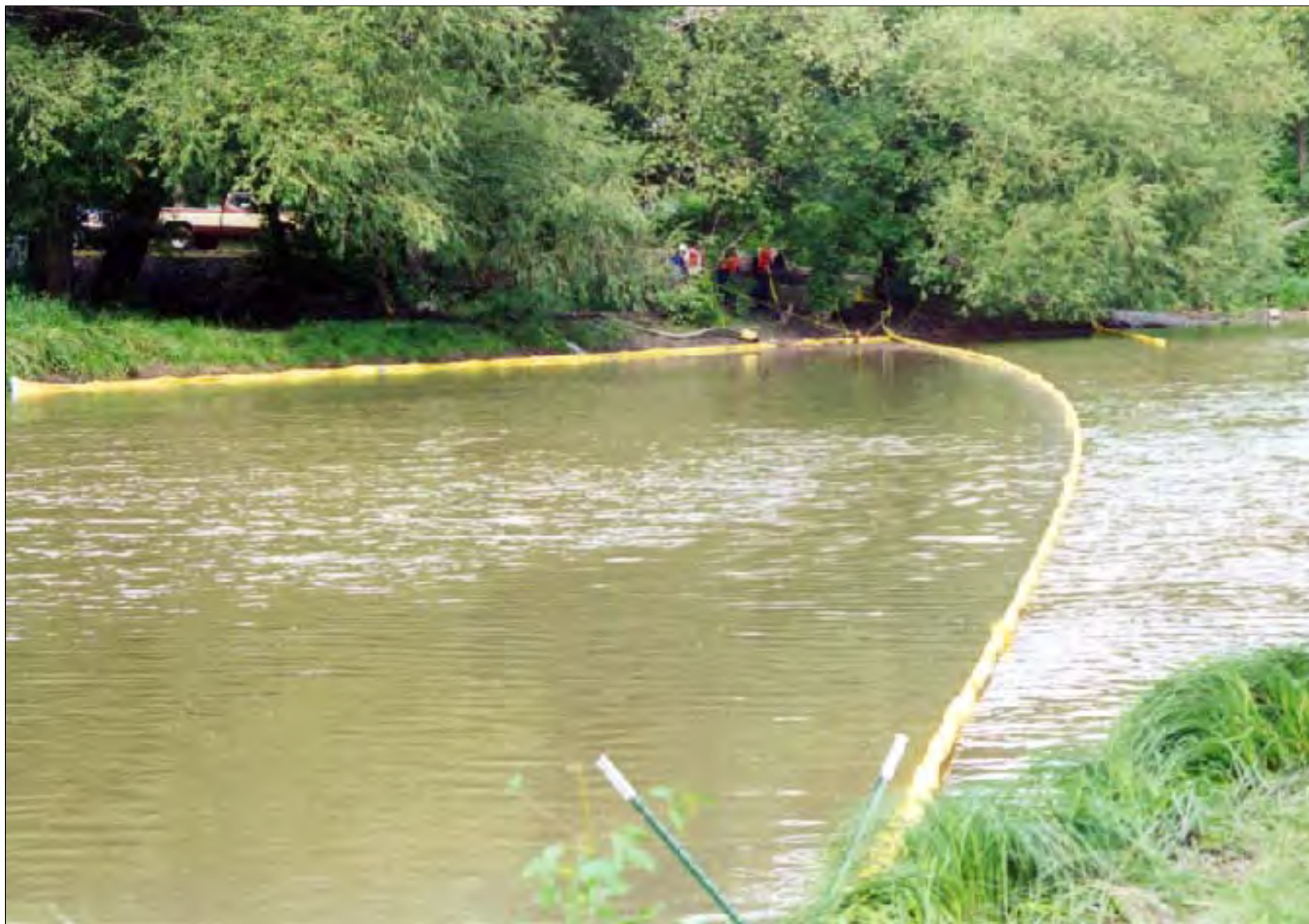
Single Diversion Boom Deployment with Shoreline Protection Red River of the North - Fargo, North Dakota
