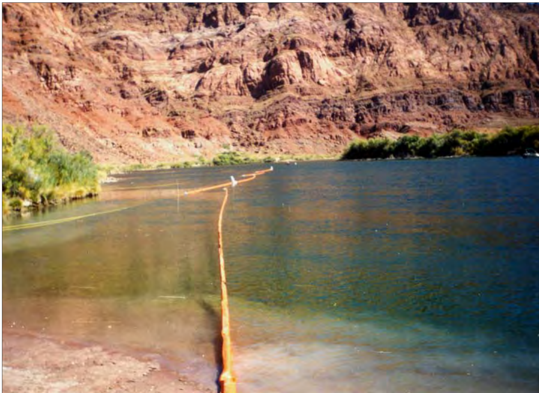
Buoy to Bank Rope Anchor System - Permanent Anchor Placement Colorado River - Page, Arizona
