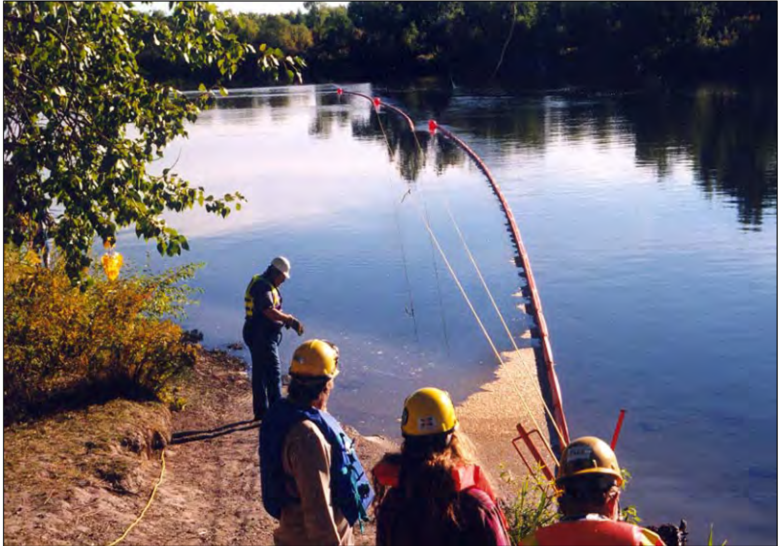
Cascade Diversionary Boom Deployment Missouri River - Great Falls, Montana
