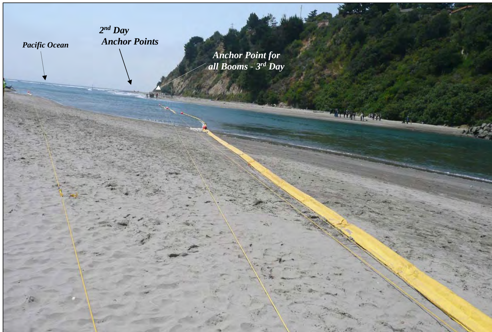
Four Booms Deployed Boom 1 Onshore due to Low Tide in Anticipation of Incoming High Tide
