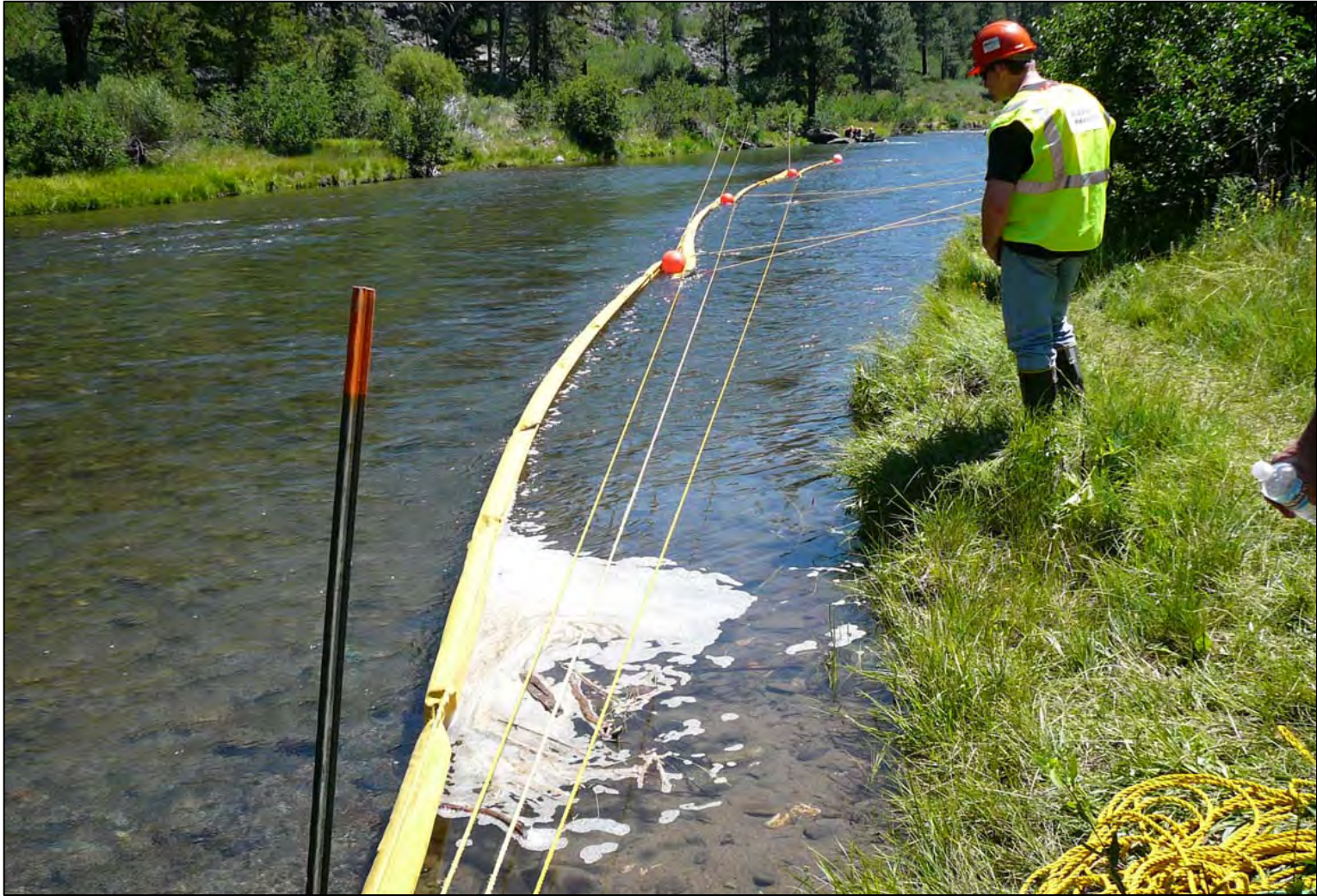
Cascade Diversionary Boom Deployment Truckee River - Truckee, CA
