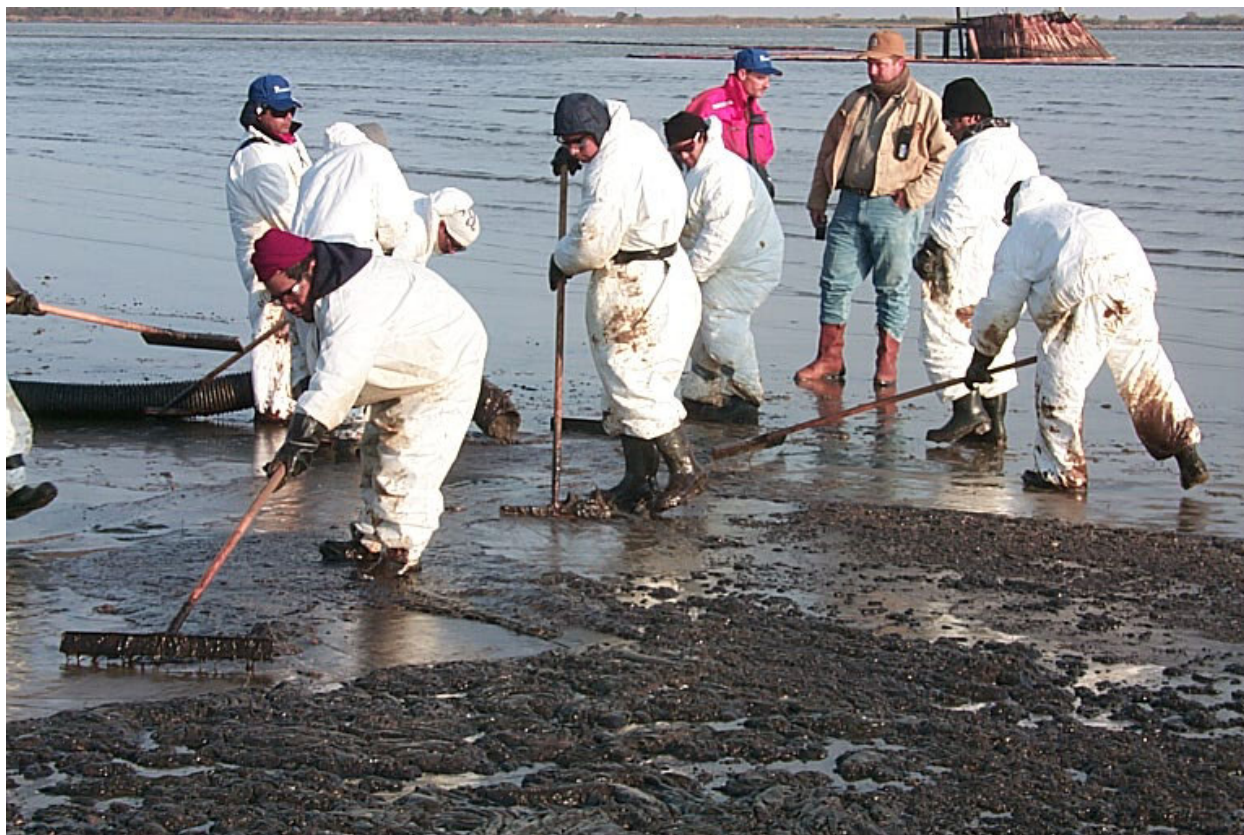
Figure 3. Cleanup of the viscous oil early in the morning when it was below the pour point.
