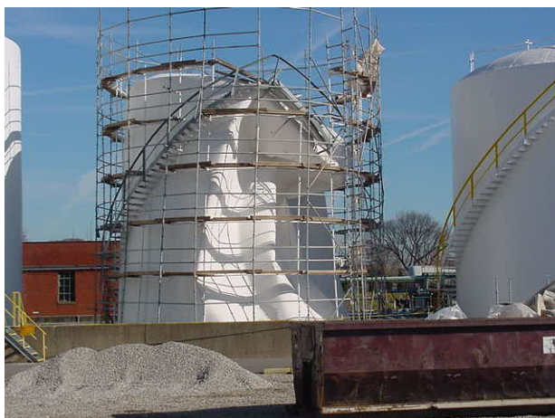
Tank Damaged Beyond Repair by Vacuum
