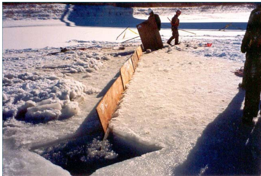
Figure 3. Diversionsary Plywood Barrier Method
