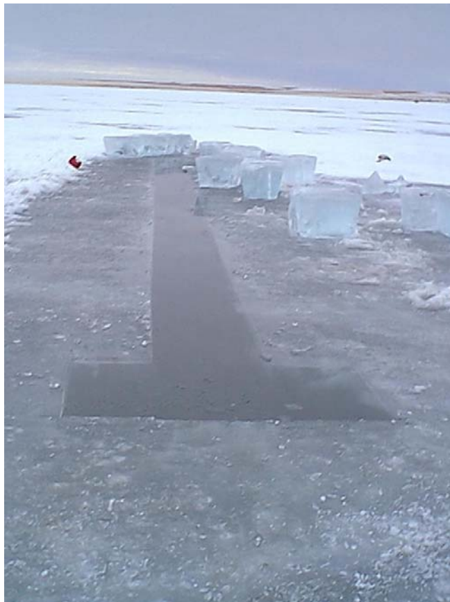
Figure 2. Slot with Recovery Sump (Approximately 50 Feet long)
