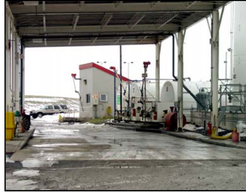
Figure 8. Depressed basin containment system. (Photograph by C&S Engineers, Inc., courtesy of Syracuse Executive Air Service, Inc.)
