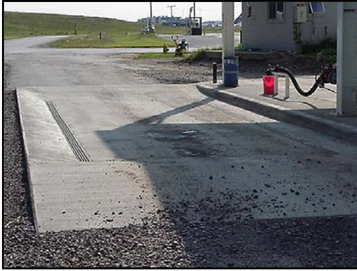
Figure 7. Depressed basin containment system. (Photograph courtesy of Syracuse Executive Air Service, Inc.)
