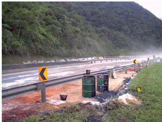
Fig. 6 – Road cleaning and decontamination.
