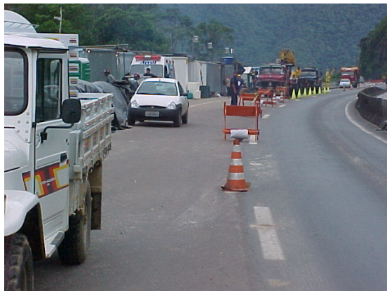
Fig. 14 – Operational base on the roadside.
