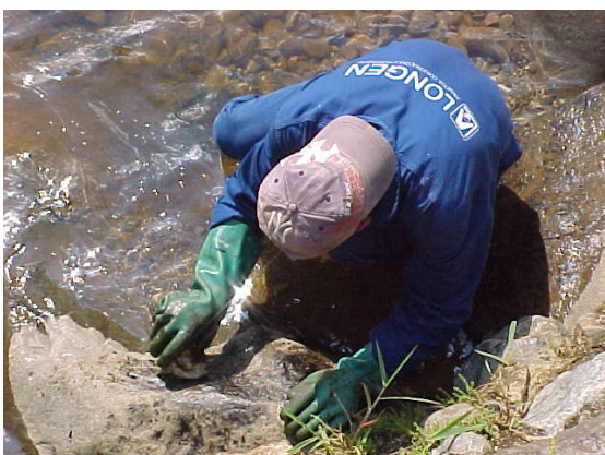
Fig 25. – Manual cleaning of river rocks.
