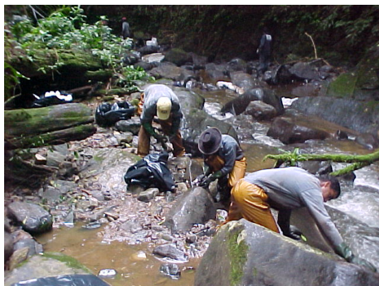
Fig. 26. – Manual cleaning of river rocks.
