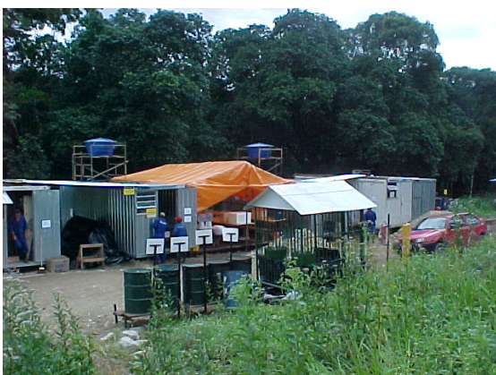
Fig. 15 – Operational base close to the river mouth.
