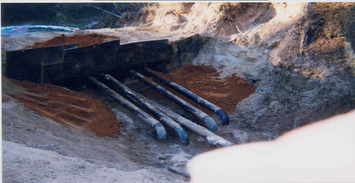
Collins, MS 12/30/99 Site: Area 1A Outfall – Underflow Pipes - Construction
