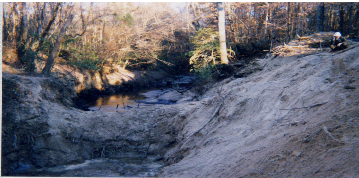
Collins, MS 12/30/99 – 12/31/99 Site: Area 1A View of Creek From Dam
