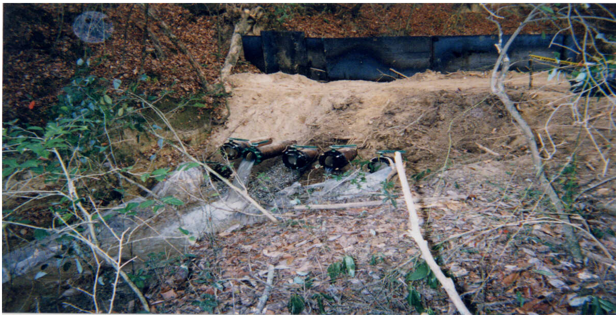
Collins, MS 12/31/99 Site: Area 1A Second Underflow Dam
