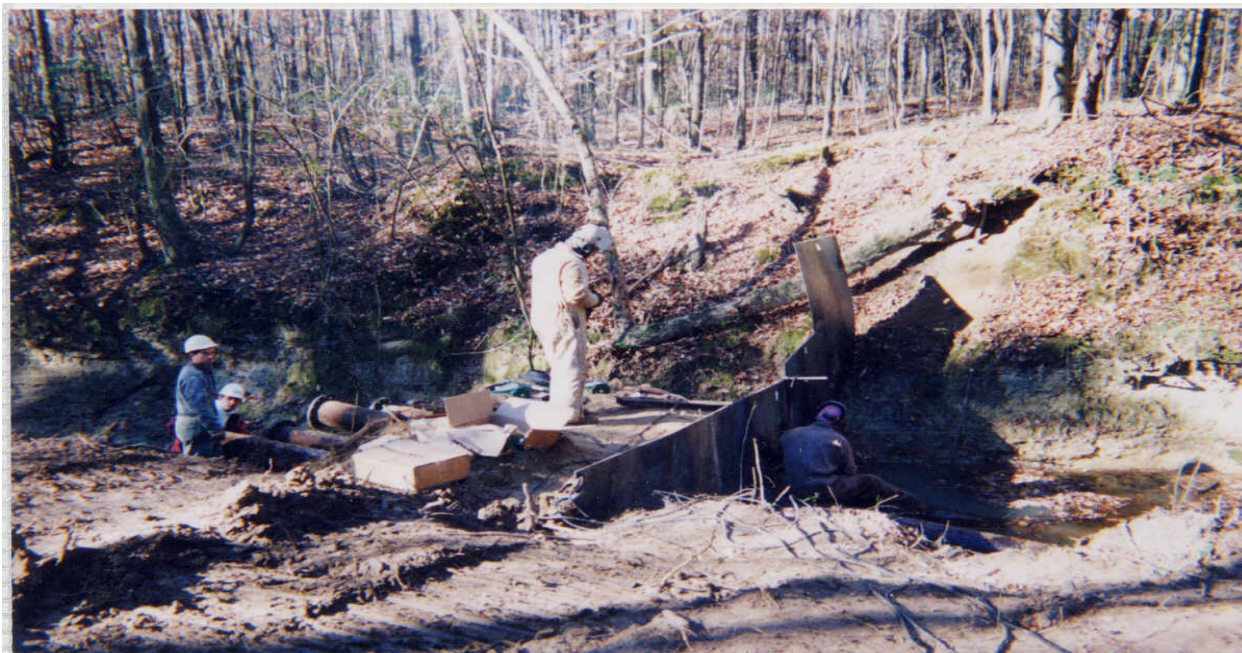
Collins, MS 12/31/99 Site: Area 1A Dam Construction
