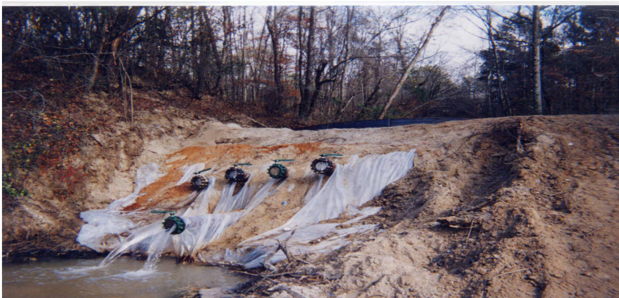
Collins, MS 01/01/00 Site: Area 1A Dam 3 Outfalls – Underflow Pipes
