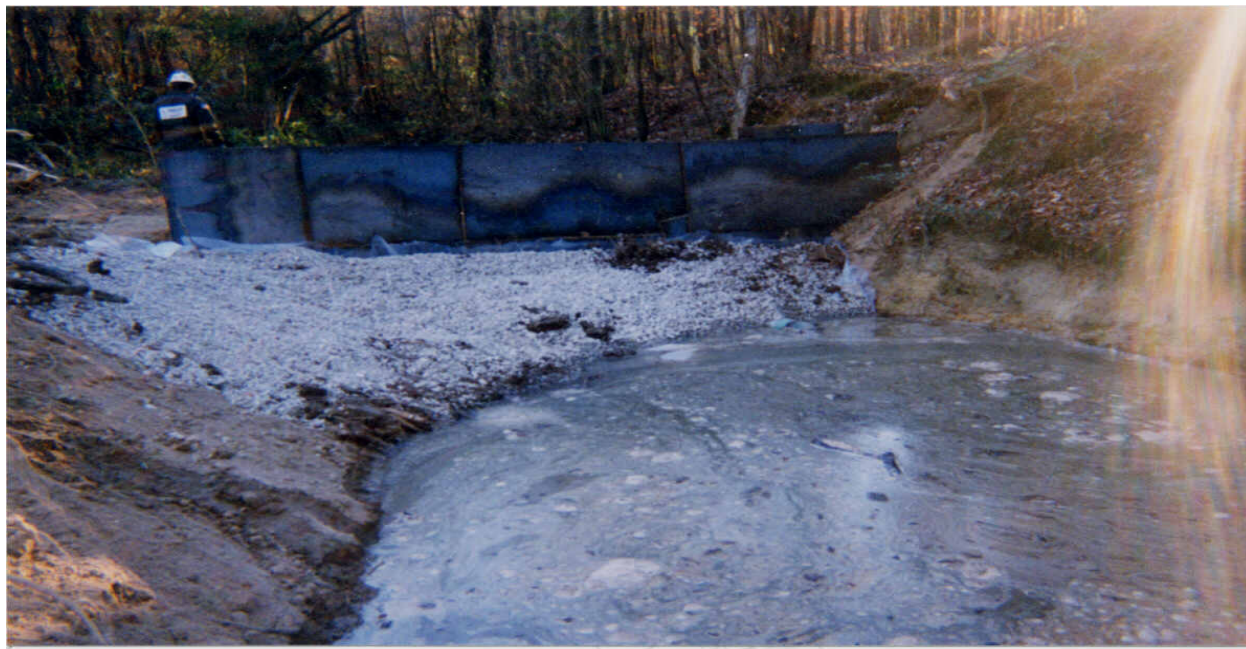
Collins, MS 12/30/99 – 12/31/99 Site: Area 1A Dam Construction
