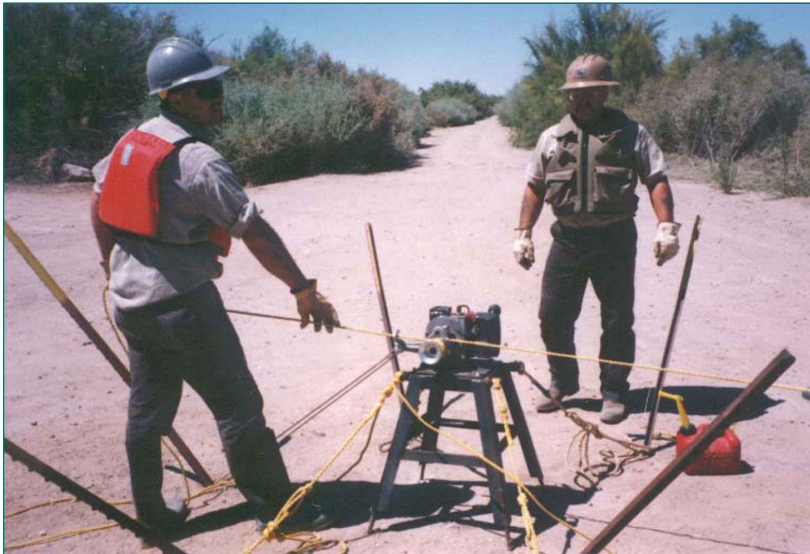
Bridge to Bank Rope Anchor System Power Wench with Rope Lead thru "D" Ring located on Bridge Column Colorado River - California
