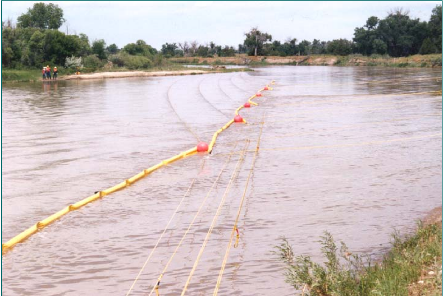
Bank to Bank Rope Anchor System North Platt River - Wyoming
