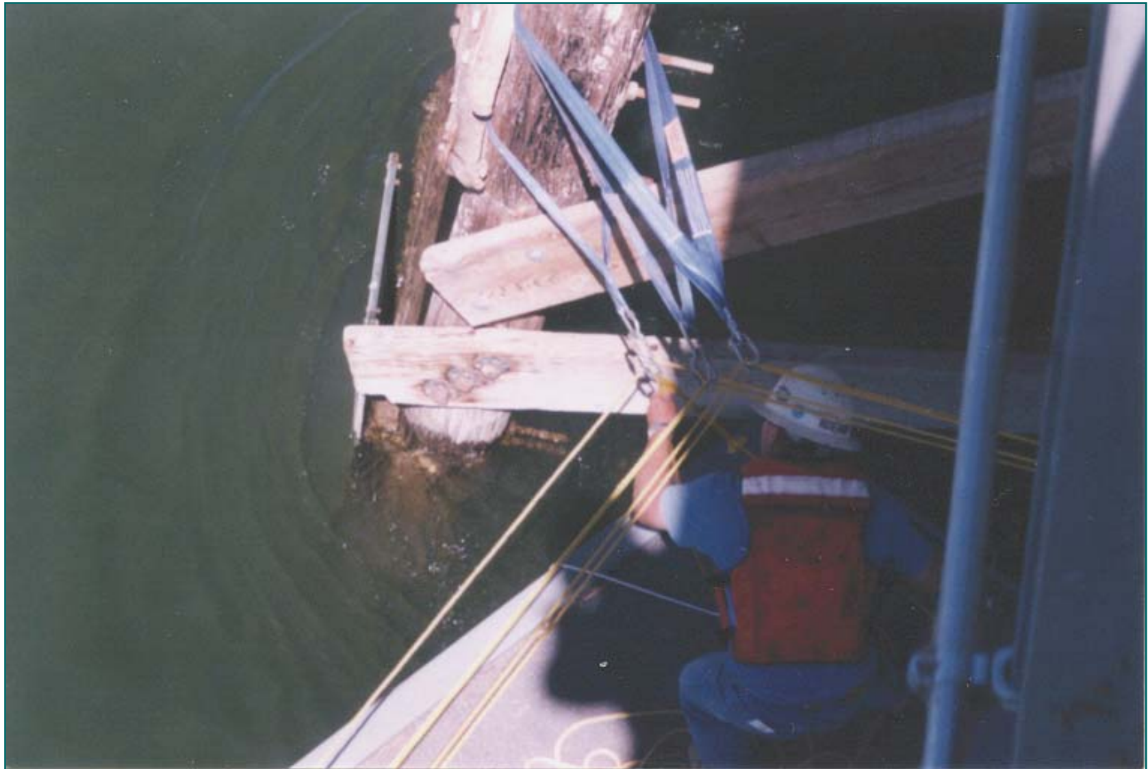
Bridge to Bank Rope Anchor System Rope Handling with Use of Webbing & "D" Rings Colorado River - California
