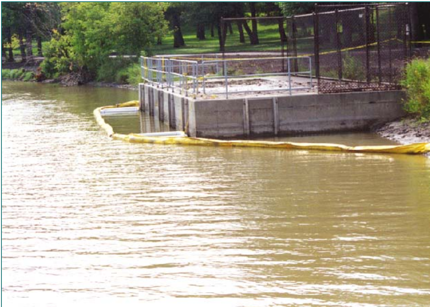
Exclusionary Boom Deployment - Water Intake with “Kim-Spacers” Red River of the North
