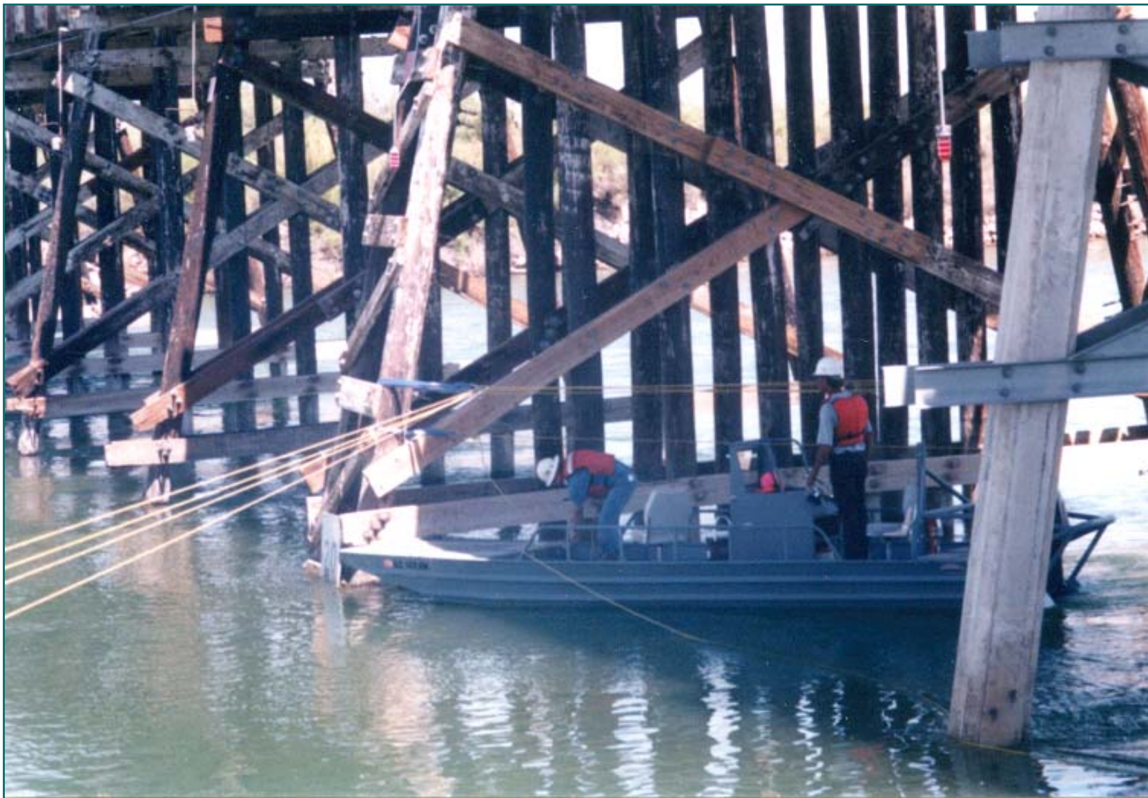
Bridge to Bank Rope Anchor System - Boat & Rope Handling Colorado River - California
