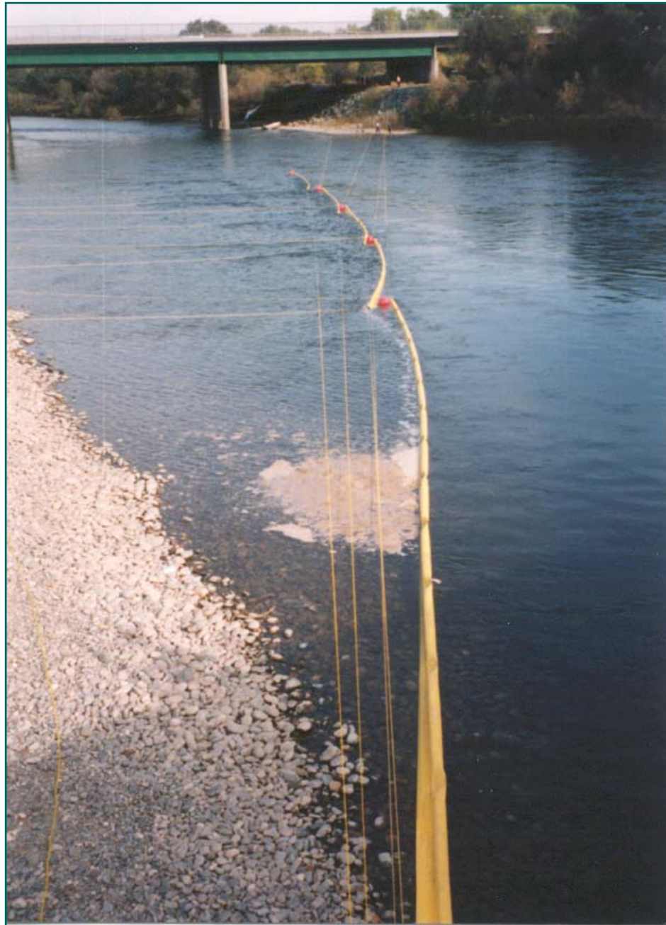
No. 4 - Boom Deployed - Bank to Bank Rope Anchor System
