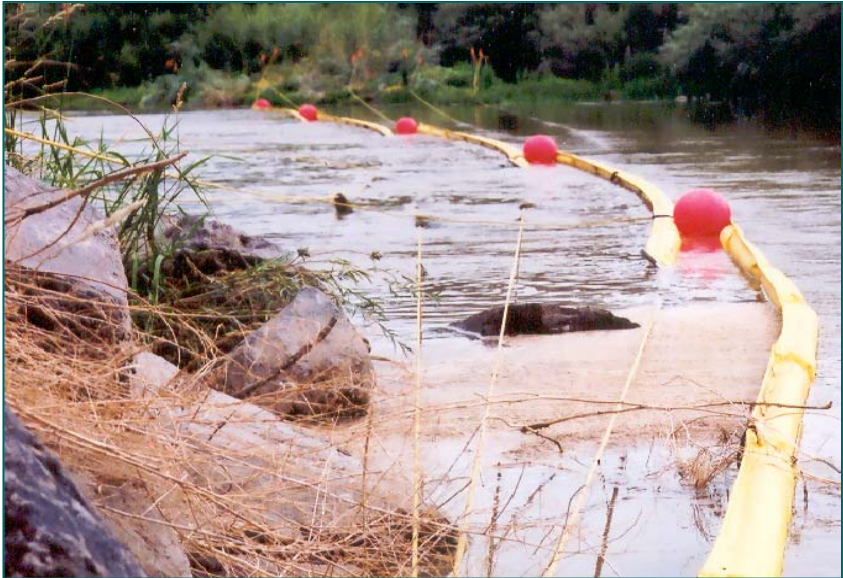
Bank to Bank Rope Anchor System Truckee River - Nevada
