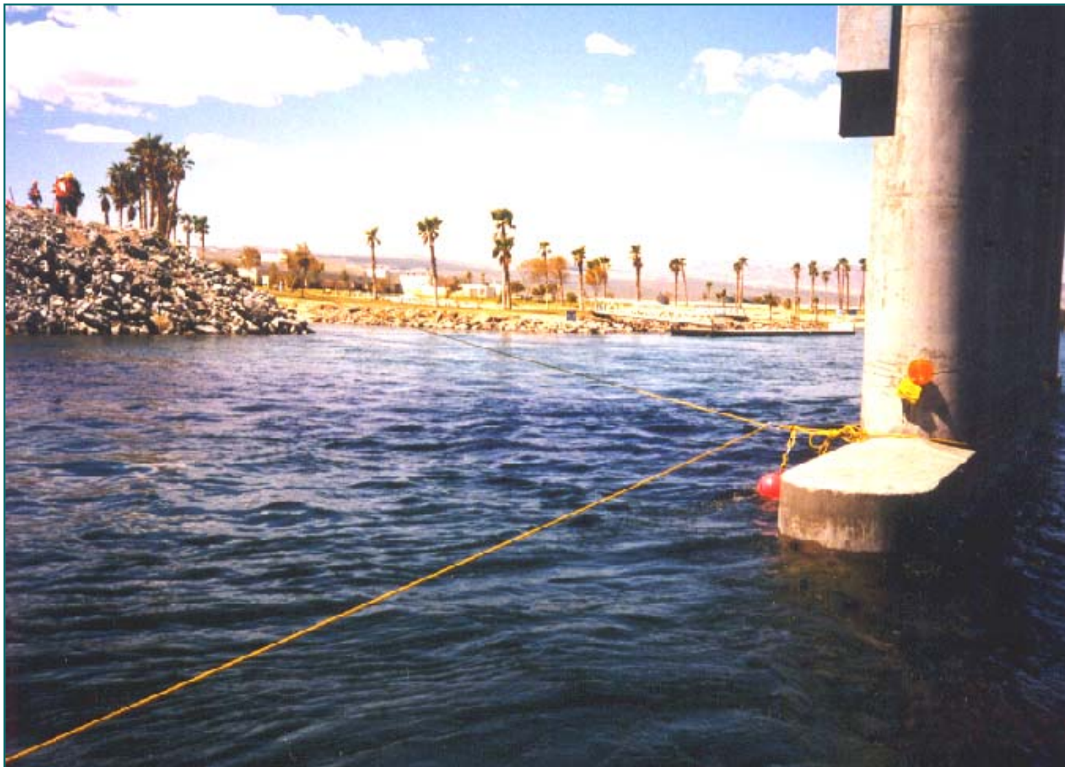
Bridge to Bank Rope Anchor System Rope Lead Anchor Collar Around Bridge Column Colorado River - Nevada
