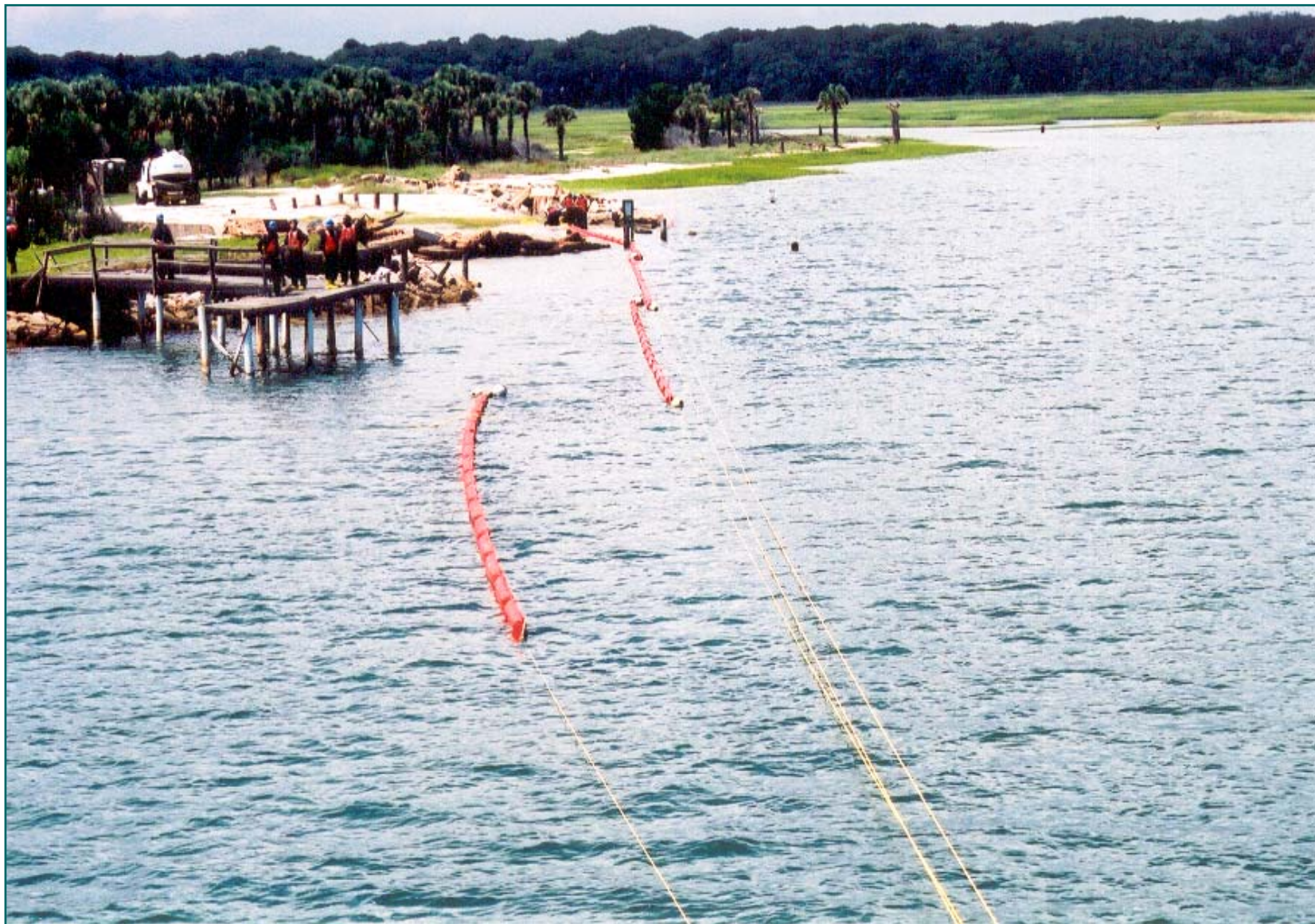
Bridge to Bank Rope Anchor System St. Johns River - Florida
