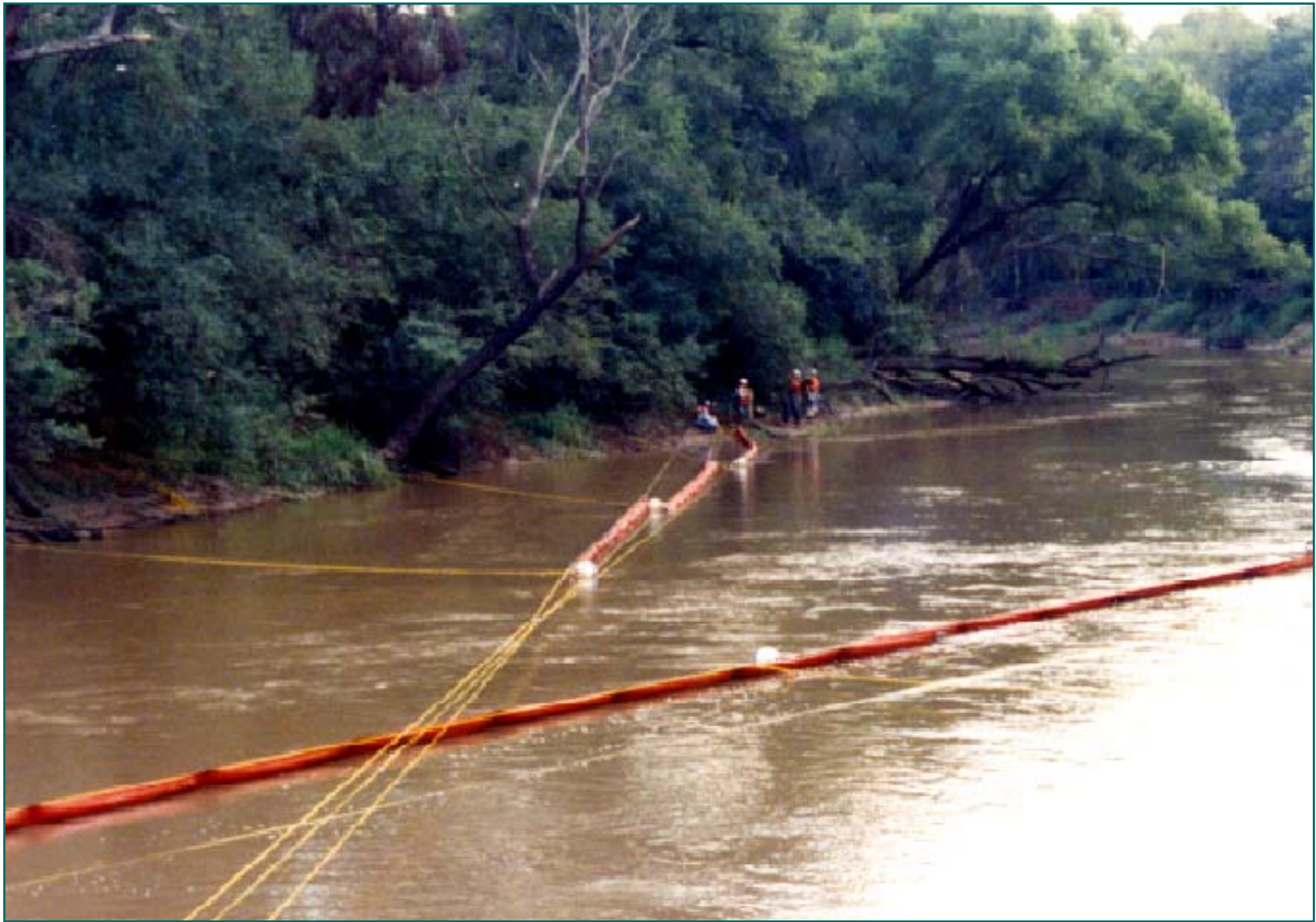
Open Cascade Chevron Diversionary Booming
