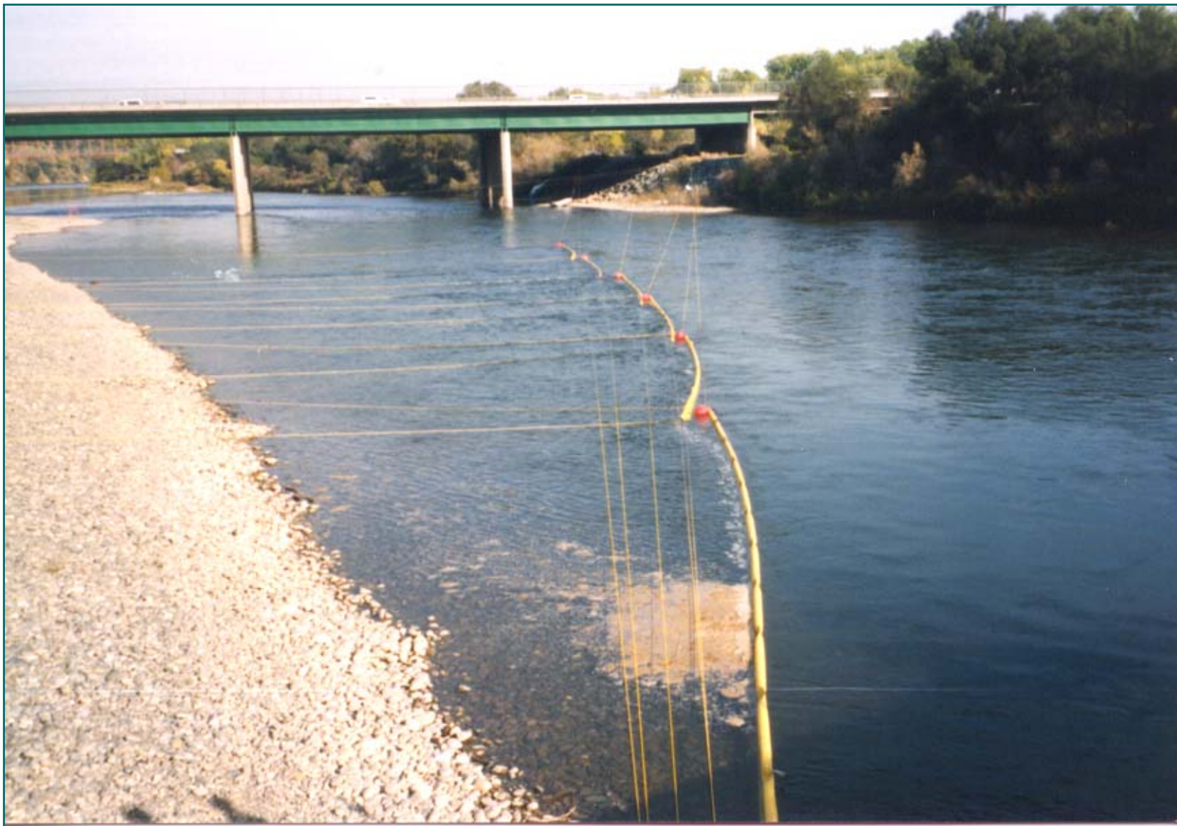
No. 6 - Boom Deployed - Bank to Bank Rope Anchor System American River - California
