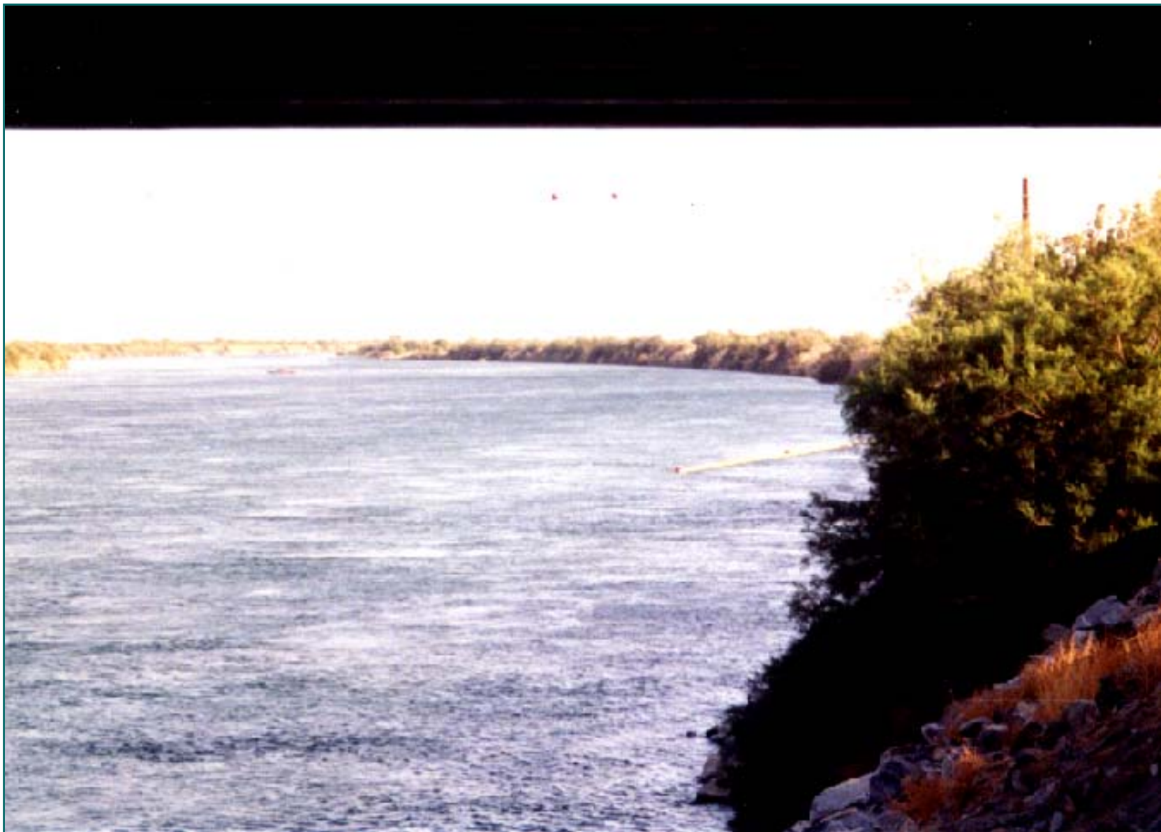
Bridge to Bank Rope Anchor System - View of Containment & Recovery Site Colorado River - Nevada
