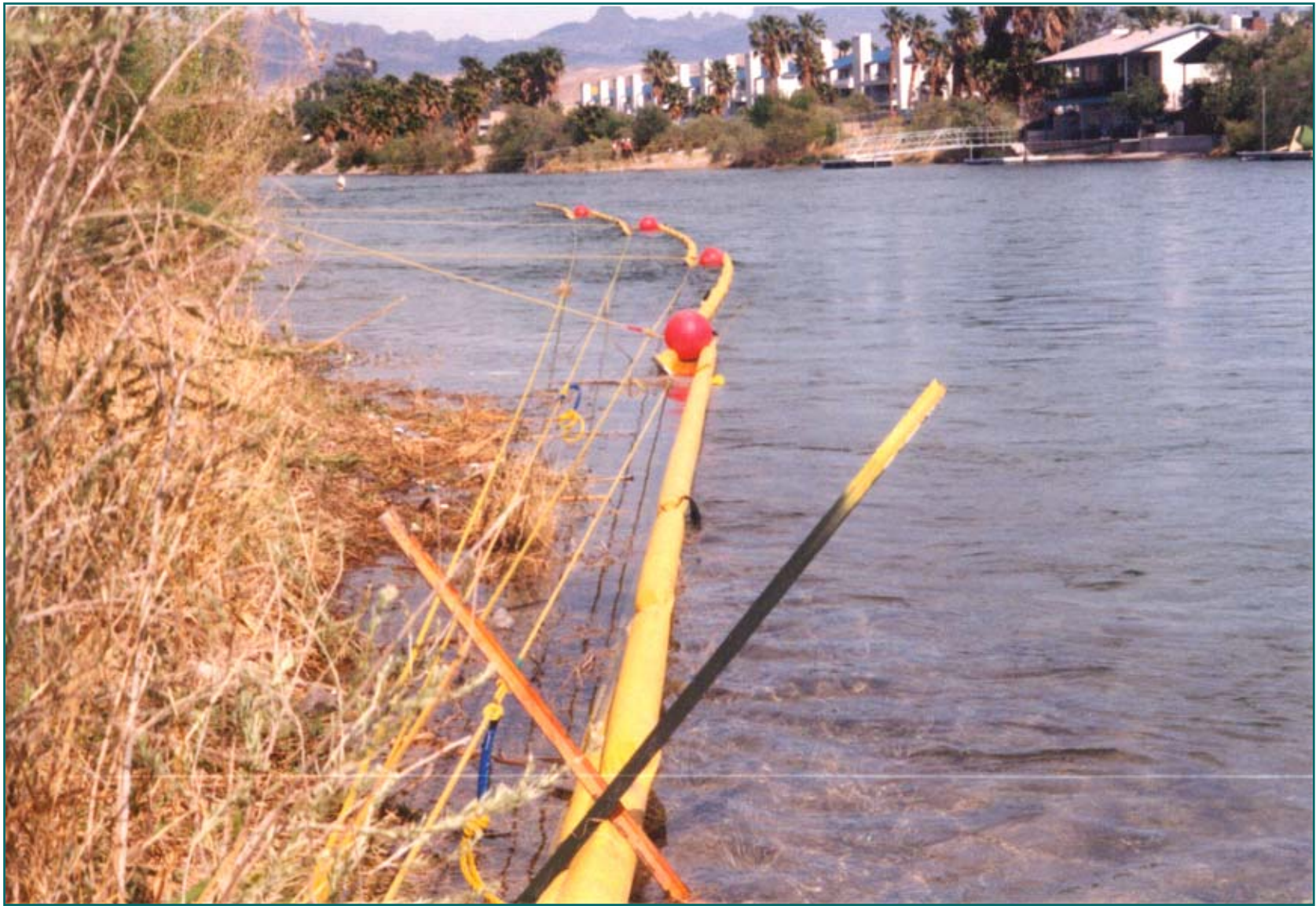
Bank to Bank Rope Anchor System Deployed Colorado River - Nevada
