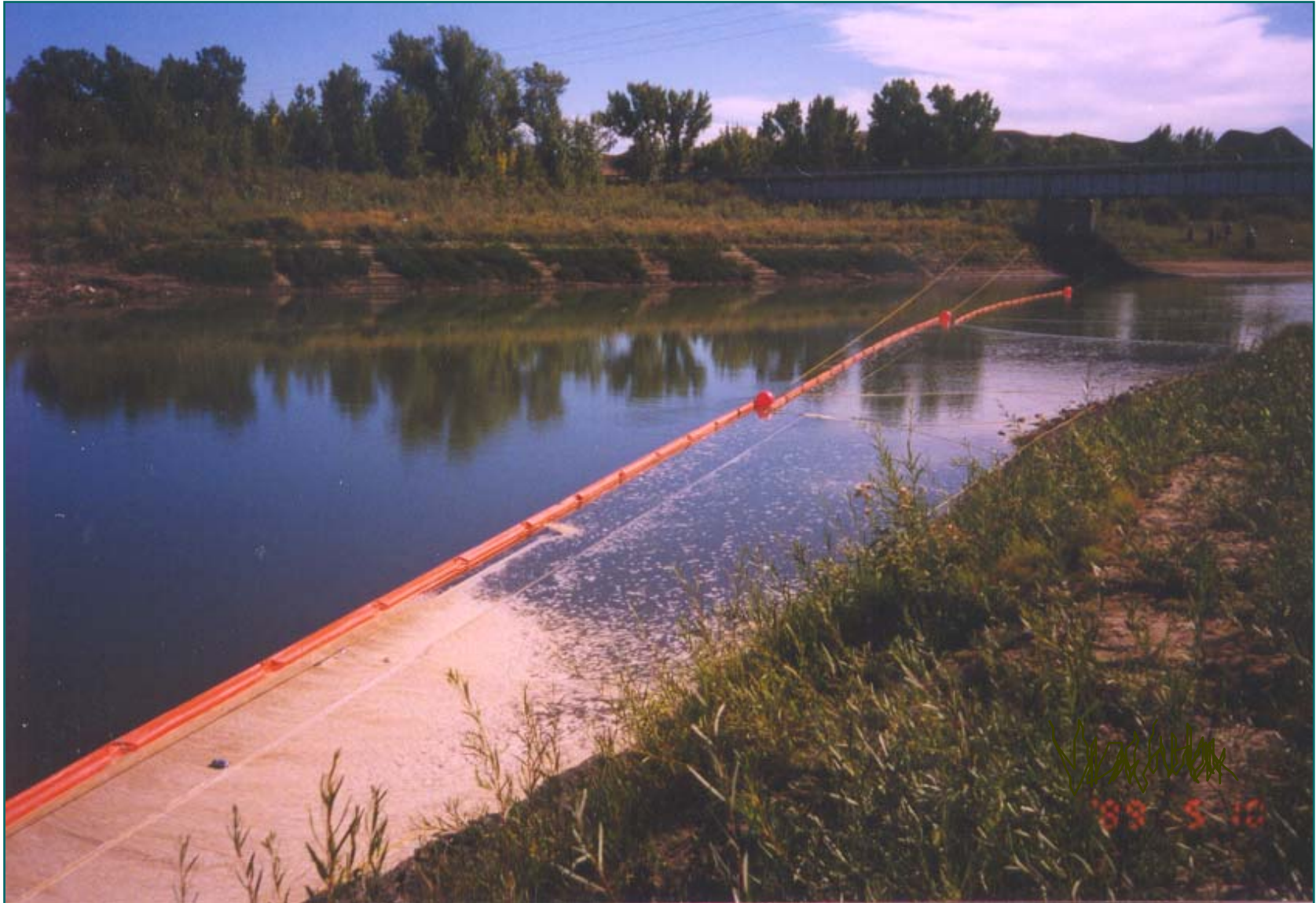
Containment Booming - River Bank Maris River - Montana
