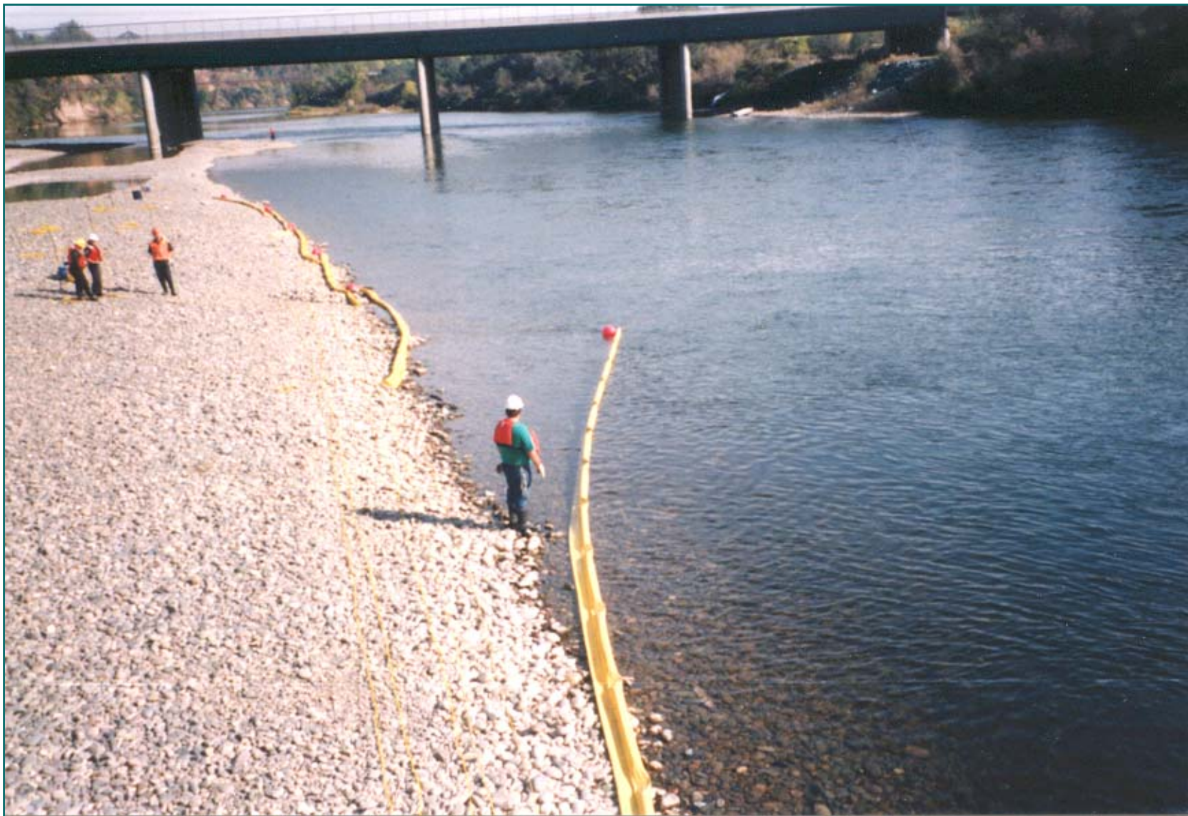
No. 1 - Boom Being Deployed - Bank to Bank Rope Anchor System American River - California
