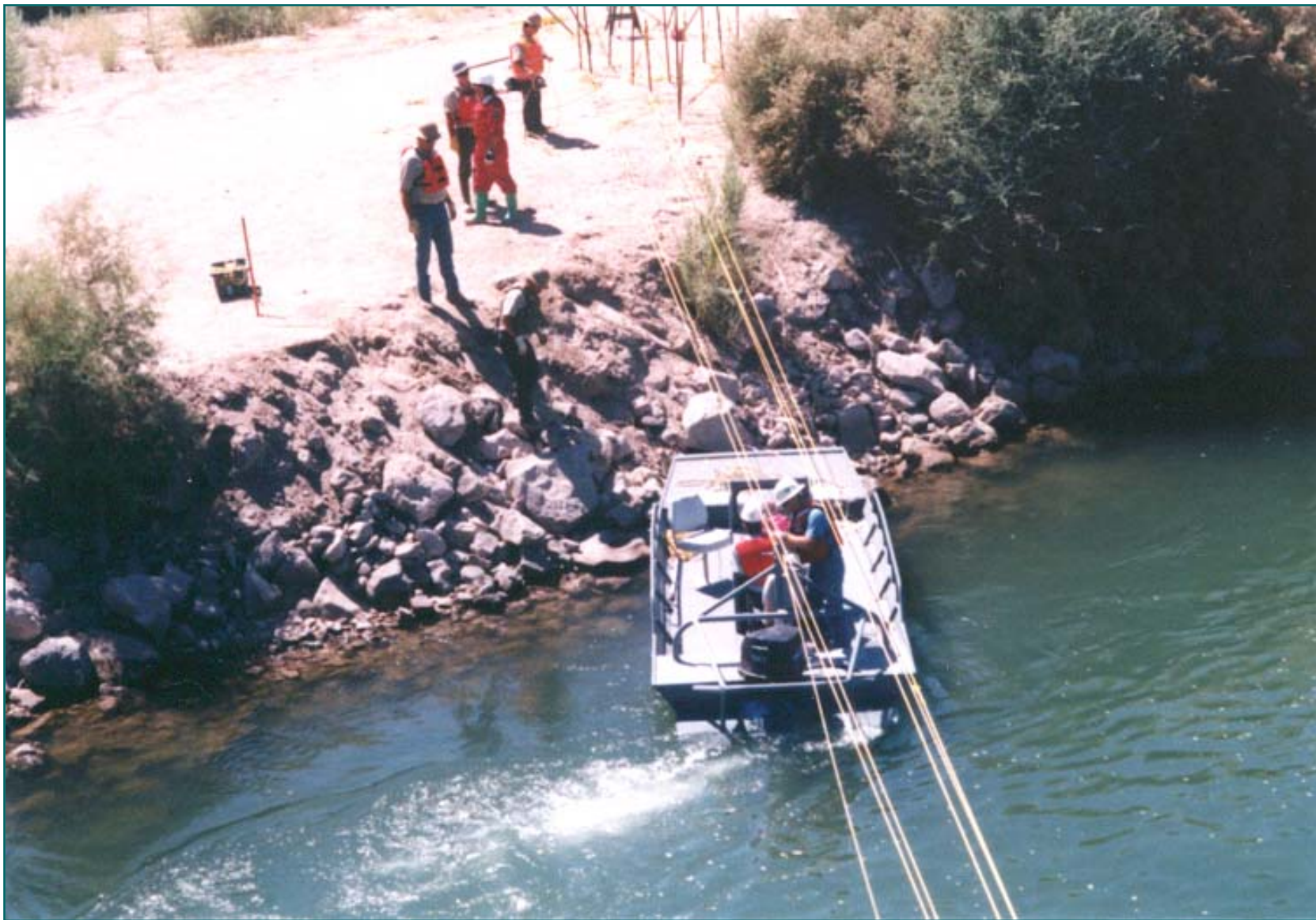
Bridge to Bank Rope Anchor System - Rope Leads to River Bank & Power Wench Colorado River - California
