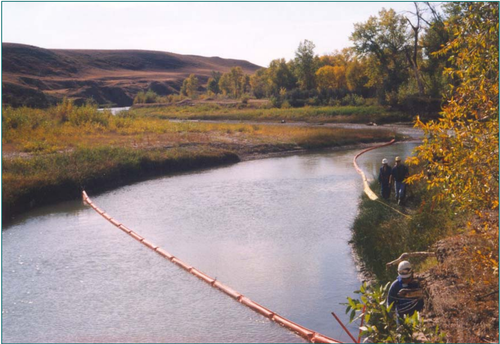
Single Diversionary Boom Deployment with Secondary Teton River - Montana
