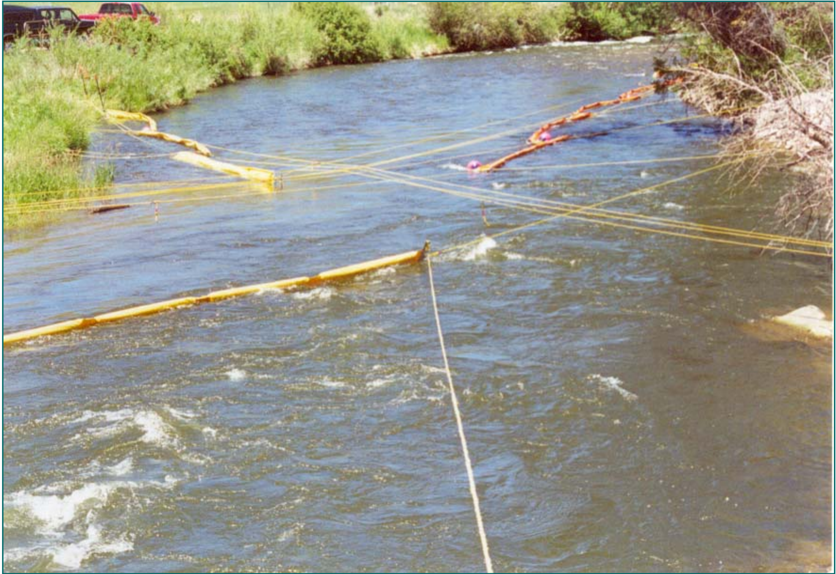
Deflection Booming - River Deployment Weber River - Utah
