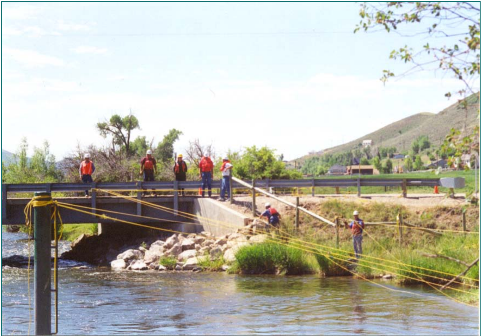
Bridge to Bank Rope Anchor System - Rope Leads Anchored to Bridge I-Beam Weber River - Utah
