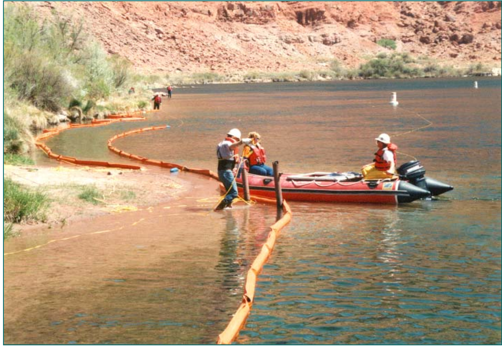
Buoy to Bank Rope Anchor System - Boom Layout on Bank Colorado River - Arizona
