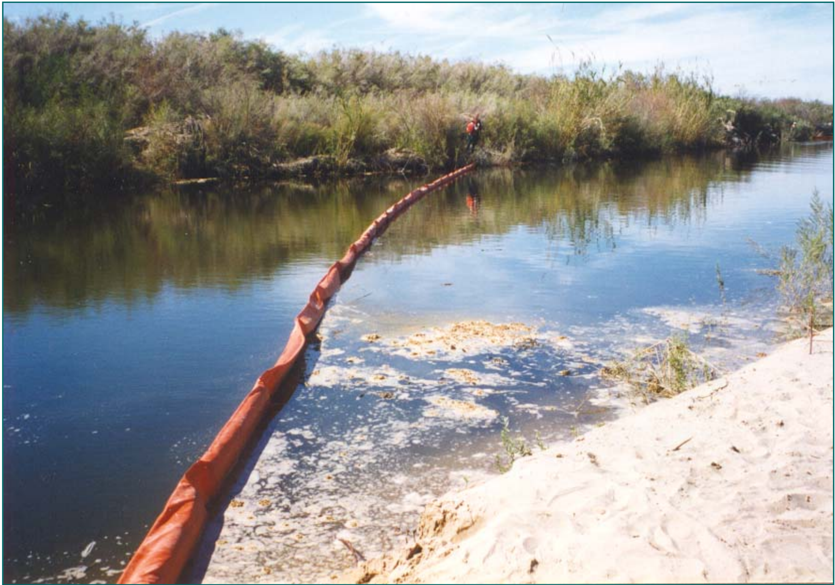
Single Diversionary/Containment Boom Deployment Channel Off of Colorado River - Arizona
