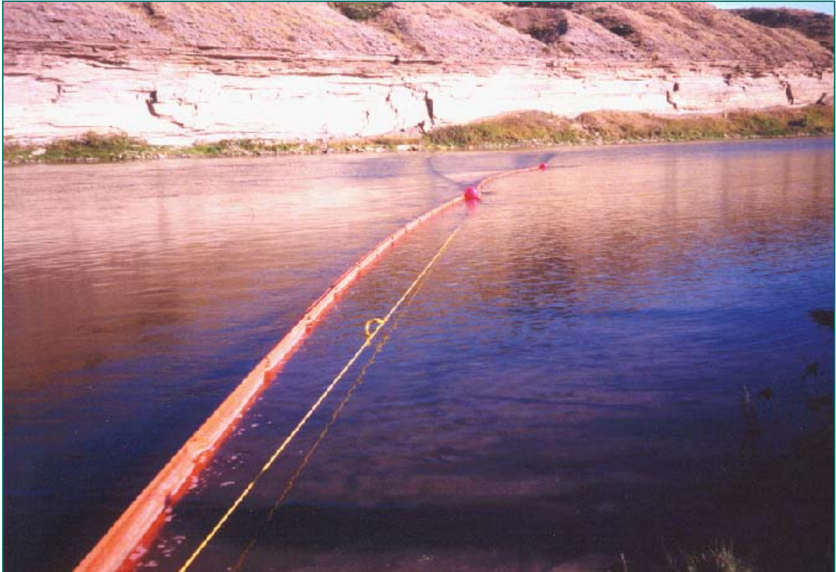
Bank to Bank Rope Anchor System Maris River - Montana
