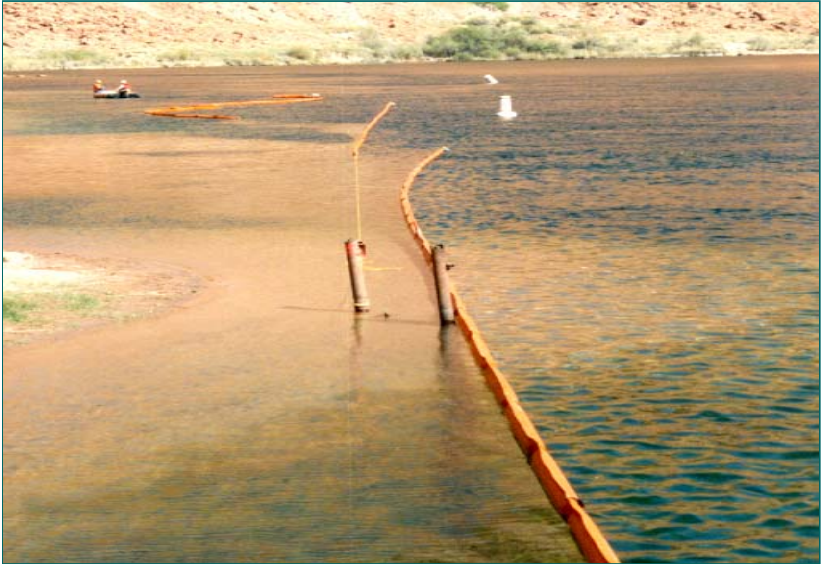
Buoy to Bank Rope Anchor System Colorado River - Arizona
