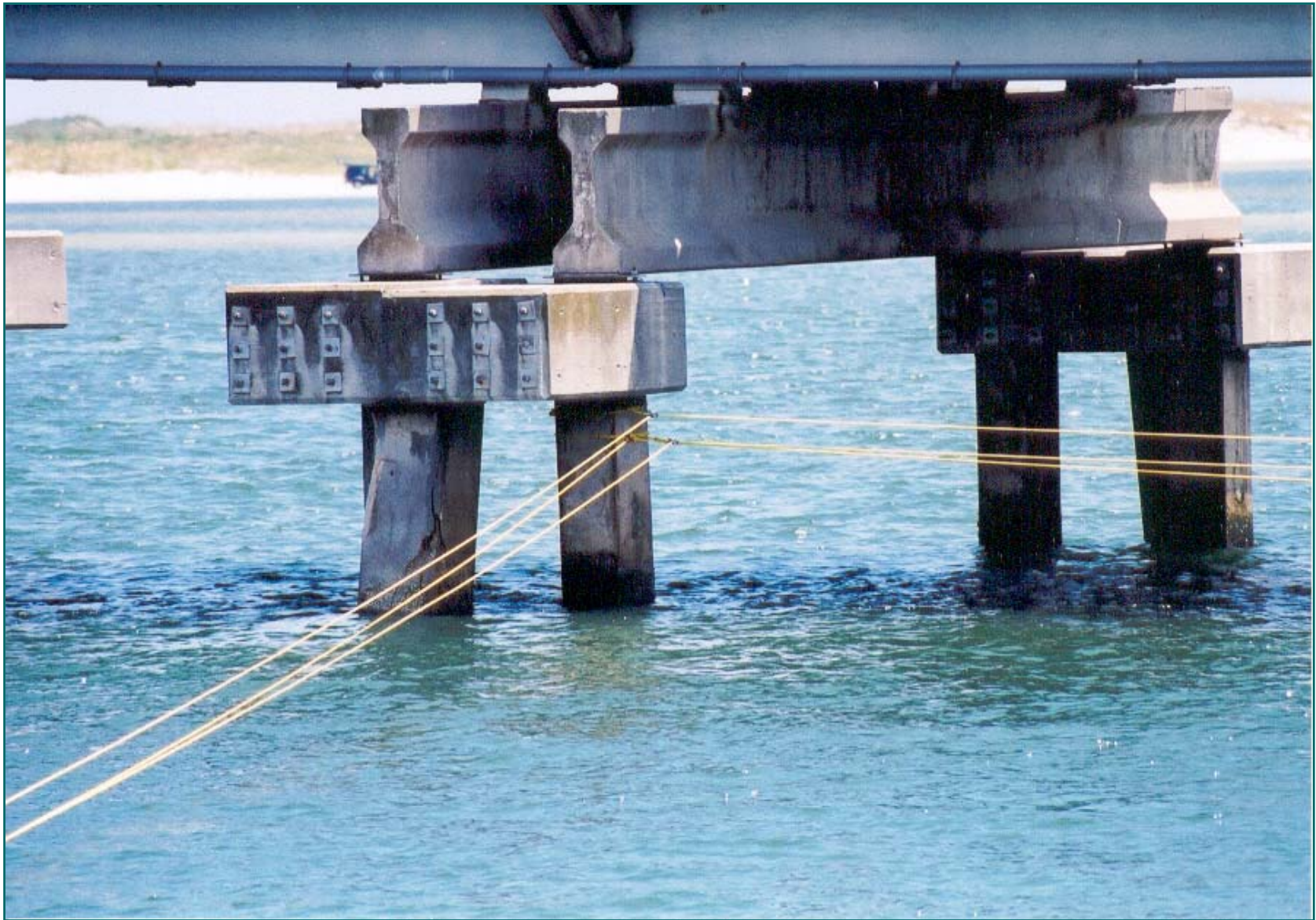
Cascade Diversionary Booming Bridge to Bank Rope Anchor System
