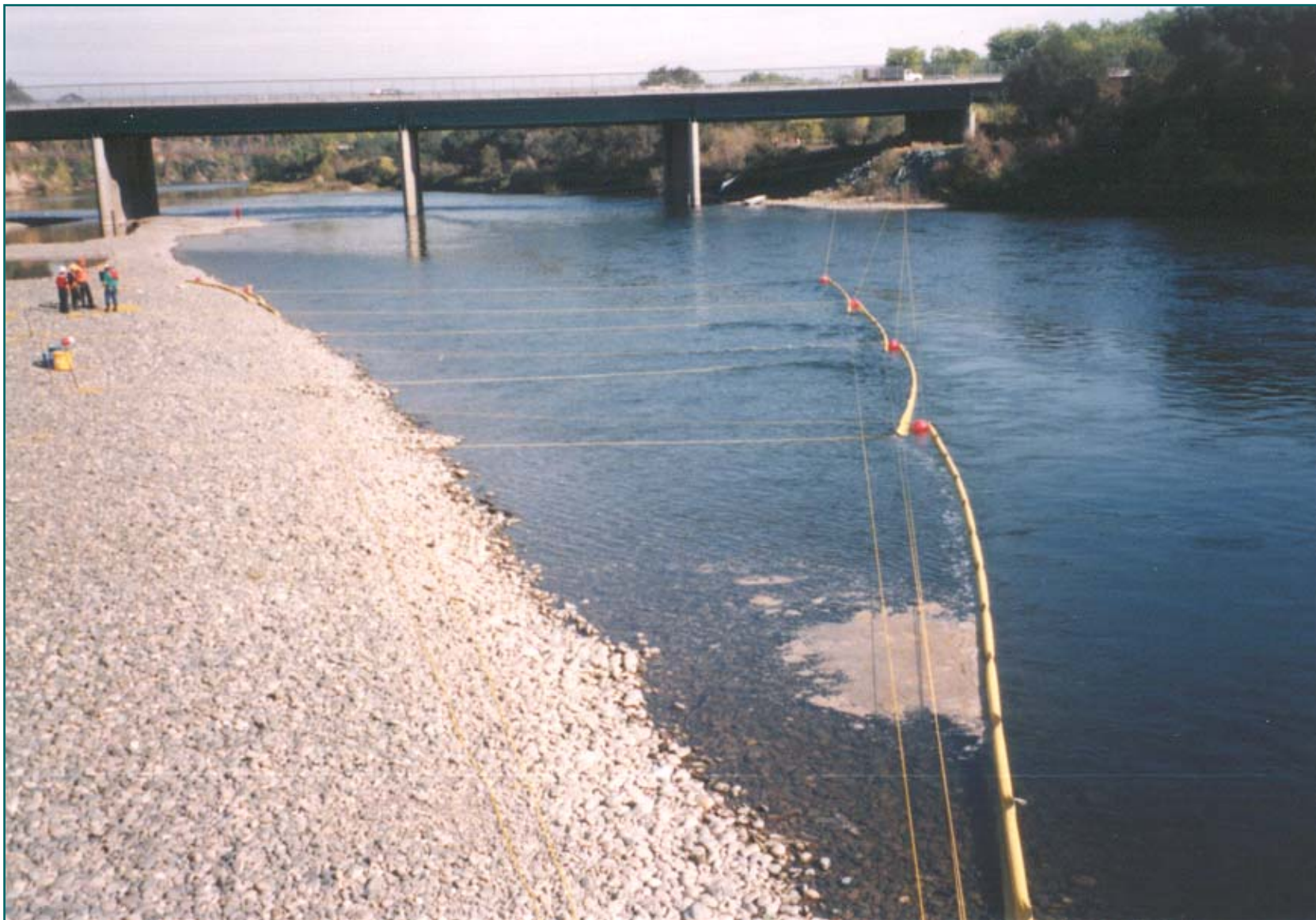
No. 4 - Boom Deployed - Bank to Bank Rope Anchor System American River - California
