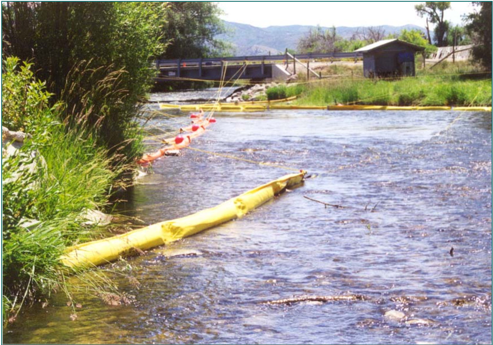
Bridge to Bank Rope Anchor System - View of Bridge Rope Anchoring Weber River - Utah
