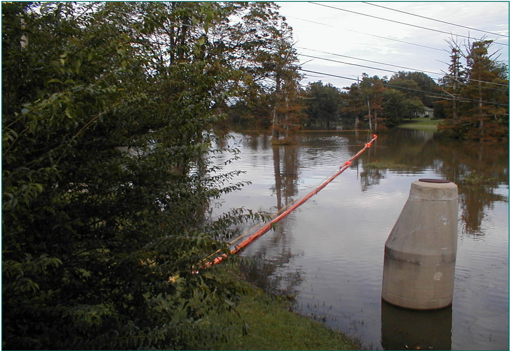
Cascade Diversionary Booming Modified Bridge to Bank Rope Anchor System (Trees)
