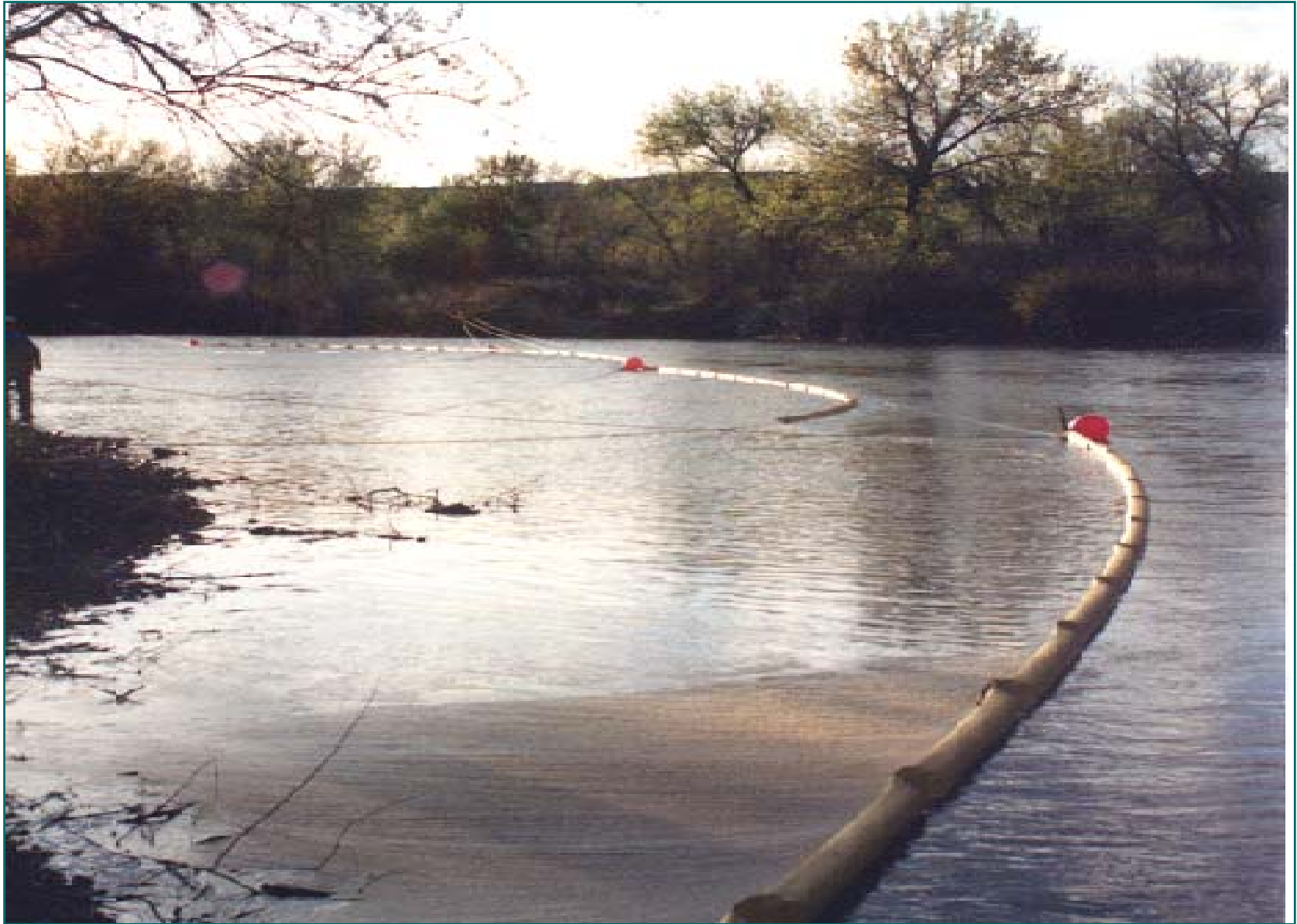
Bank to Bank Rope Anchor System Arkansas River - Colorado
