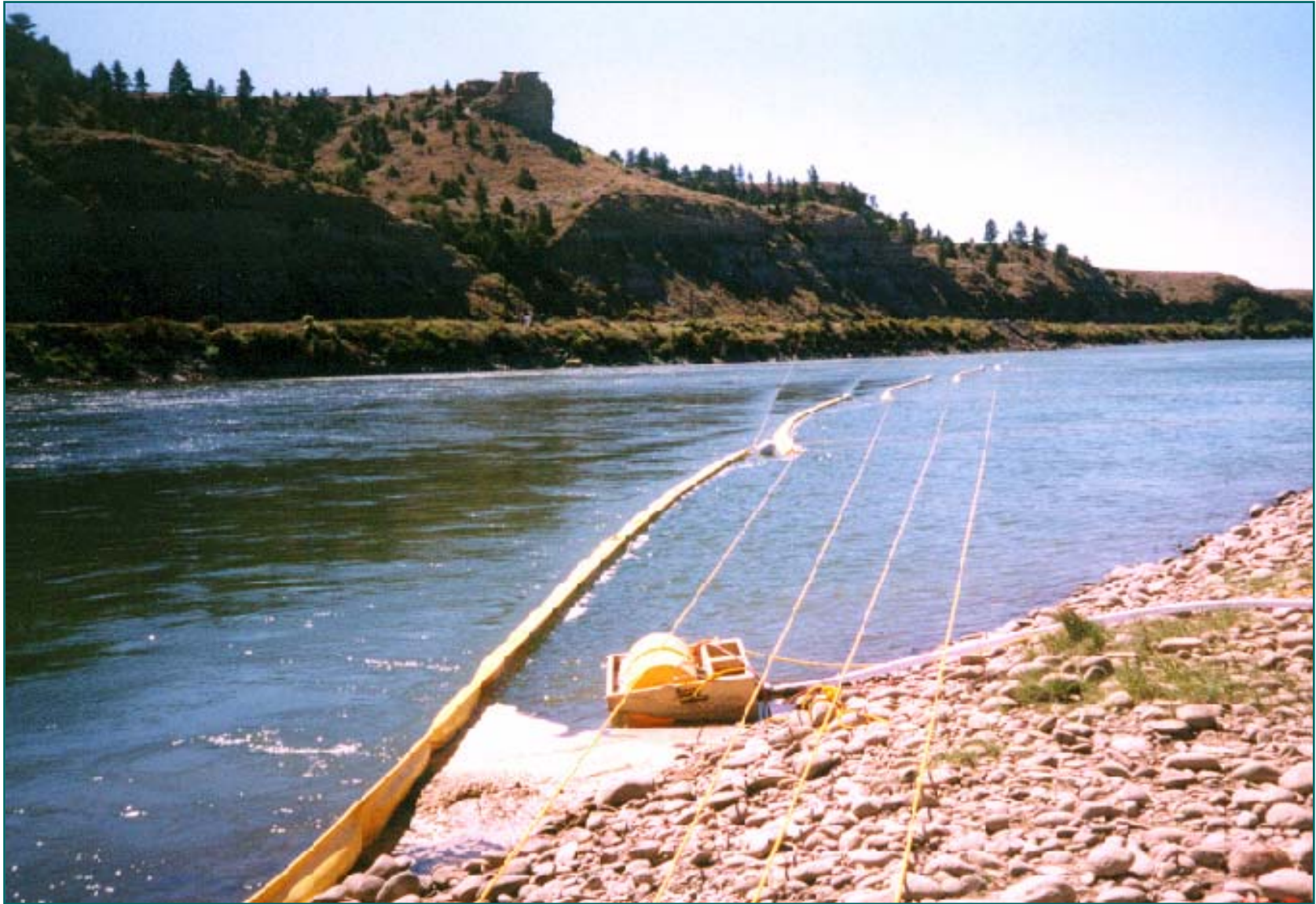
Bank to Bank Rope Anchor System Yellow Stone River - Montana
