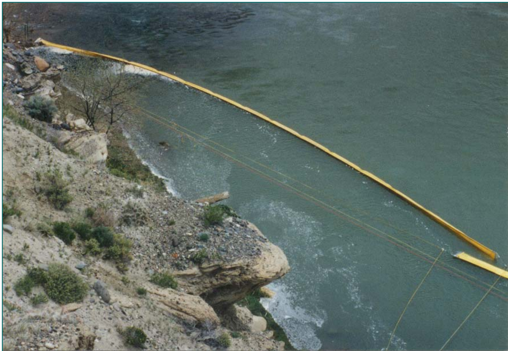
Containment Booming – Cascade System Shoshone River - Wyoming
