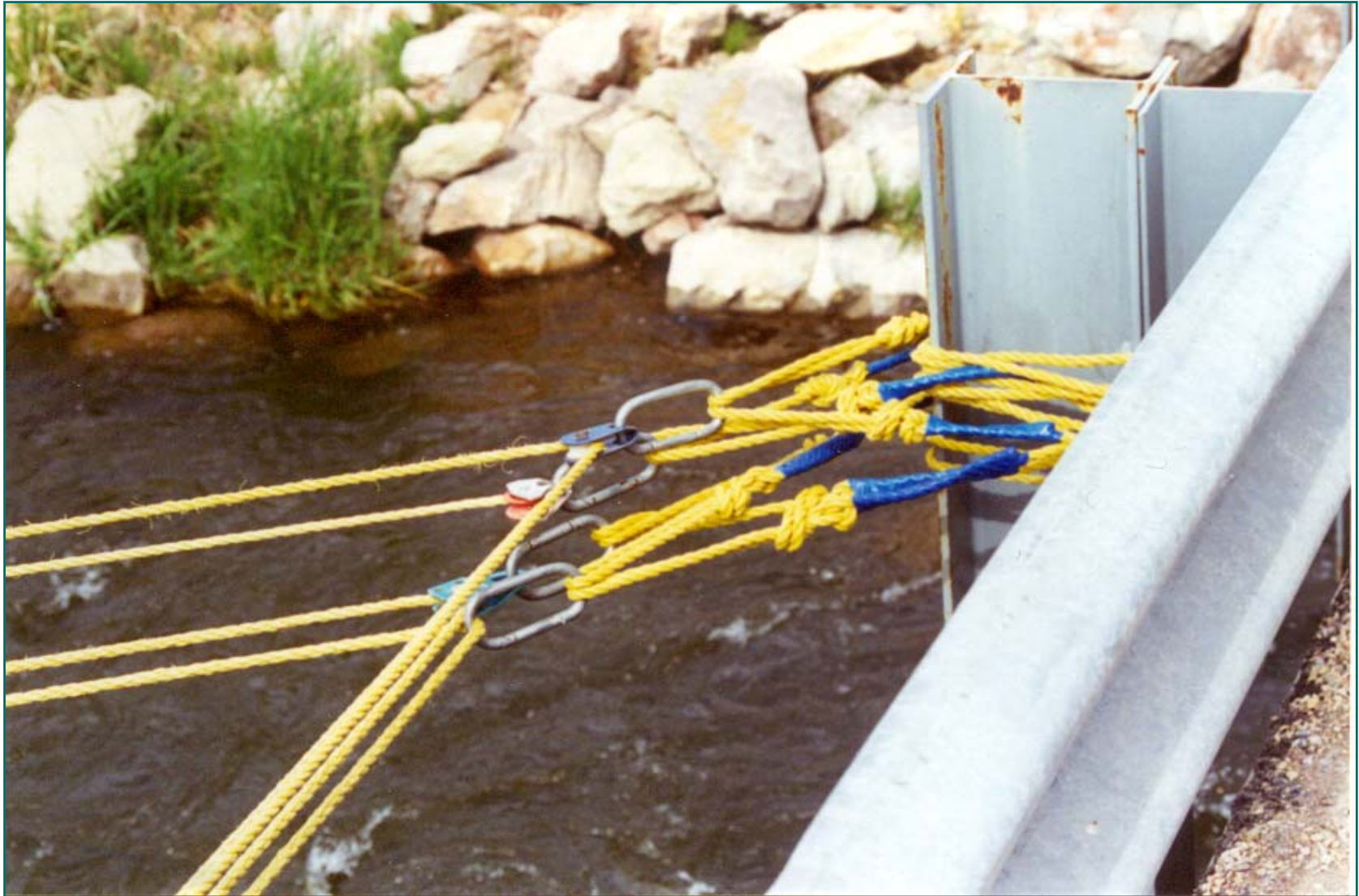
Bridge to Bank Rope Anchor System Rope Leads with Pulleys Anchored to Bridge I-Beam Weber River - Utah
