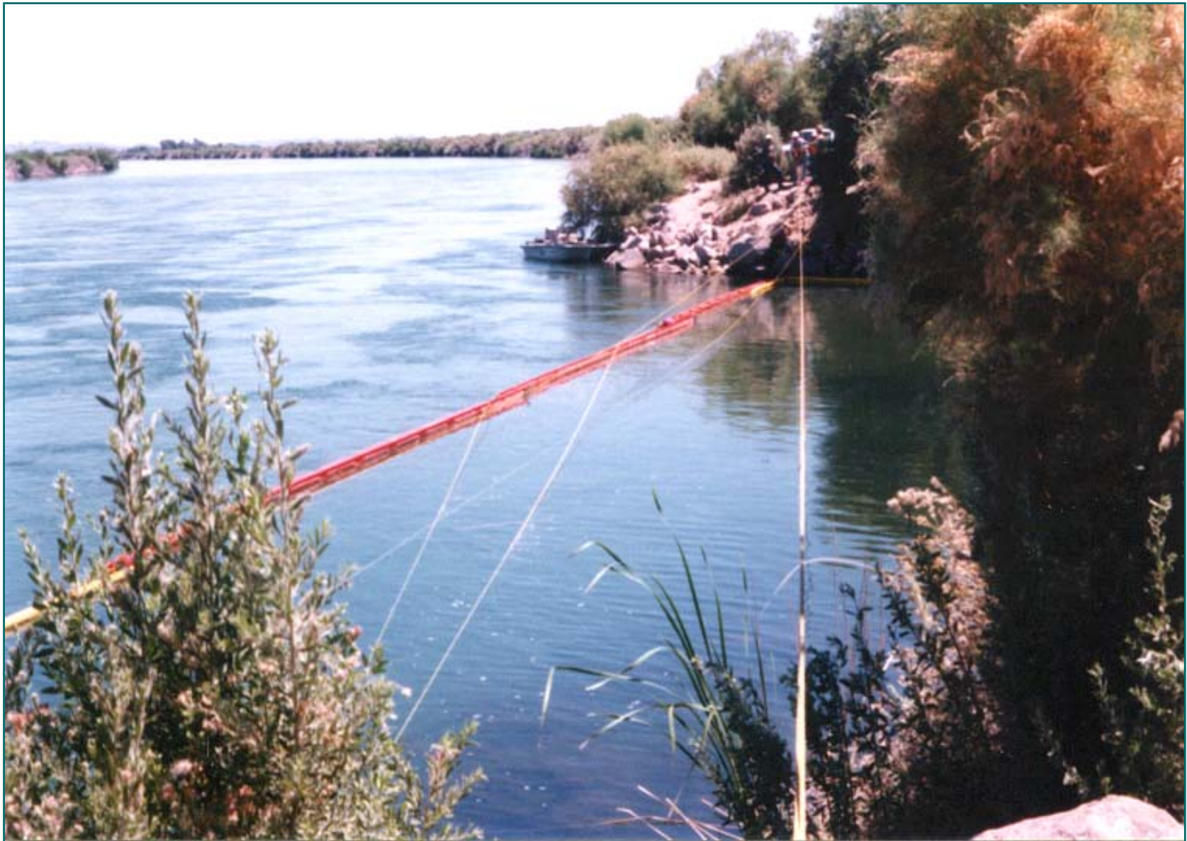
Bridge to Bank Rope Anchor System - Containment Area Colorado River - California
