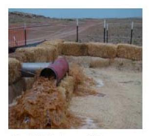
The initial release of the hydrostatic test water into the straw bale dewatering structure.
