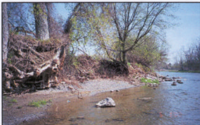
Streambank before treatment, Summer 2000.
