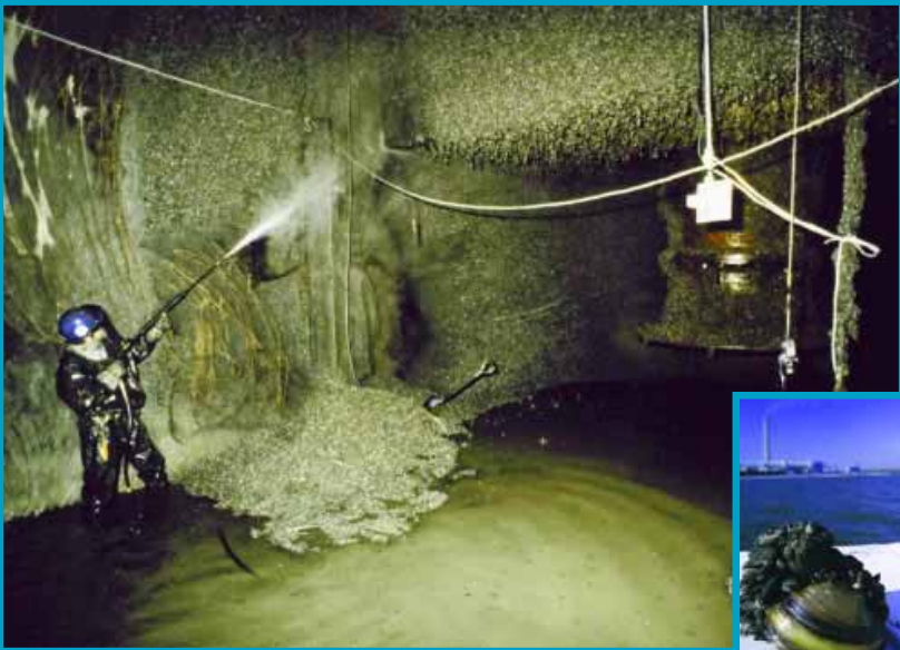
Workers remove zebra mussels from a water intake pipe at DTE Energy's Monroe Power Plant
