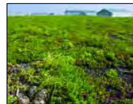
A killdeer ( Charadrius vociferous ) nest of eggs is spotted on the 10.4-acre living green roof at Ford Motor Company's Ford Rouge Center in Dearborn, Michigan. The roof is constructed of a bioengineered stormwater management system that includes drought tolerant sedum and a recycled fabric growing medium. Many innovative solutions have been put into place at the Ford Rouge Center to manage the flow of water on the property in a way that is beneficial to the environment. The use of porous pavement, buffer strips and living green roofs all help to filter and clean stormwater run-off helping protect water quality and providing wildlife habitat.
