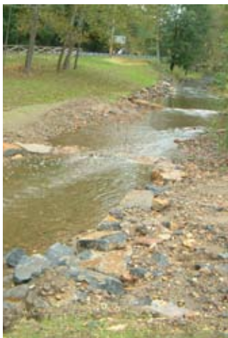
At top, existing debris; above and left, examples of grade control
