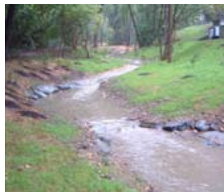
At top, existing debris; above and left, examples of grade control
