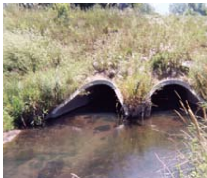
At right, Glenside culvert; above and below, culverts created for improved fish passage
