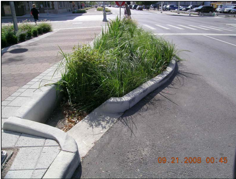
Small bioswale located in a curb cut.. Runoff from the road surface enters the curb cut in the foreground, and is filtered through the soil and vegetation.
