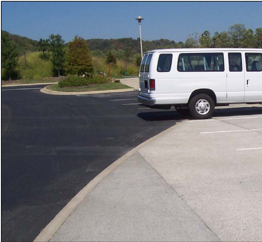
Some permeable pavement systems are indistinguishable from traditional impermeable pavement.
