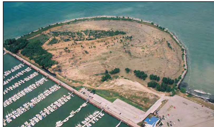
Aerial view of the Lorain Confined Disposal facility.
