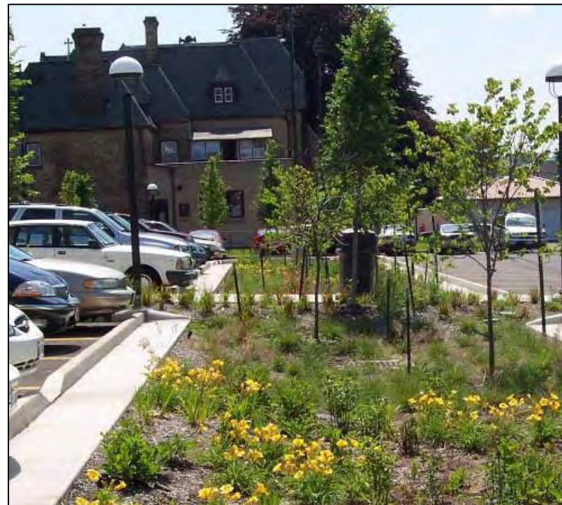
Bioswales are constructed areas filled with permeable soils and native plants, they help control and treat stormwater runoff.
