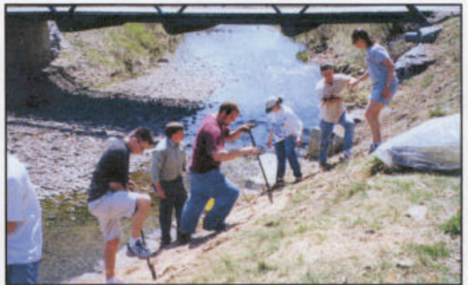
Holland High students and volunteers planting Red osier dogwood and Streamco willow bare-root seedlings through Geo-jute erosion control fabric, Spring 2001.
