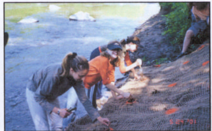
Potters Road Elementary students planting Red osier dogwood and Streamco willow bare-root seedlings through Geo-jute erosion control fabric, Spring 2001.
