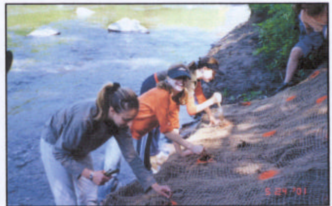
Potters Road Elementary students planting Red osier dogwood and Streamco willow bare-root seedlings through Geo-jute erosion control fabric, Spring 2001.
