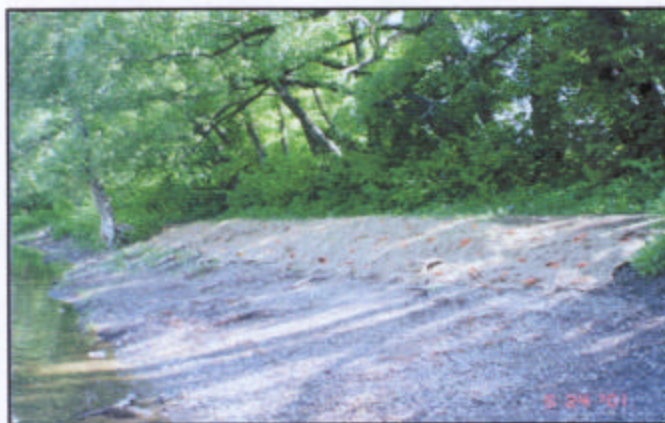
Geo-jute erosion control fabric was placed on banks before planting to aid in stabilizing soil.
