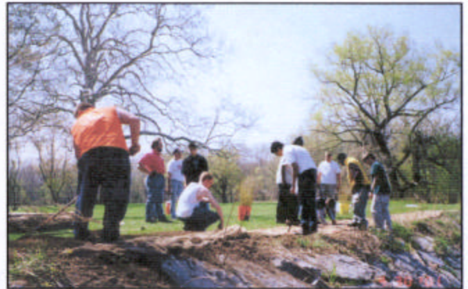
Gow School students and West Seneca AmeriCorps planting seedlings through Geo-jute erosion control fabric above the slope rock and filling in a gully (lower left), Spring 2001.
