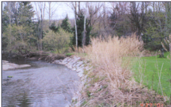
Herbaceous vegetation along bank, providing insufficient erosion control, just prior to planting with Red osier dogwood and Streamco willow bare-root seedlings, Spring 2001.
