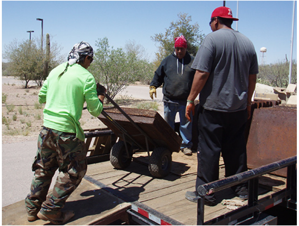
Tribal ecoAmbassador student interns transporting hardened pavers. Photo courtesy of TOCC.
