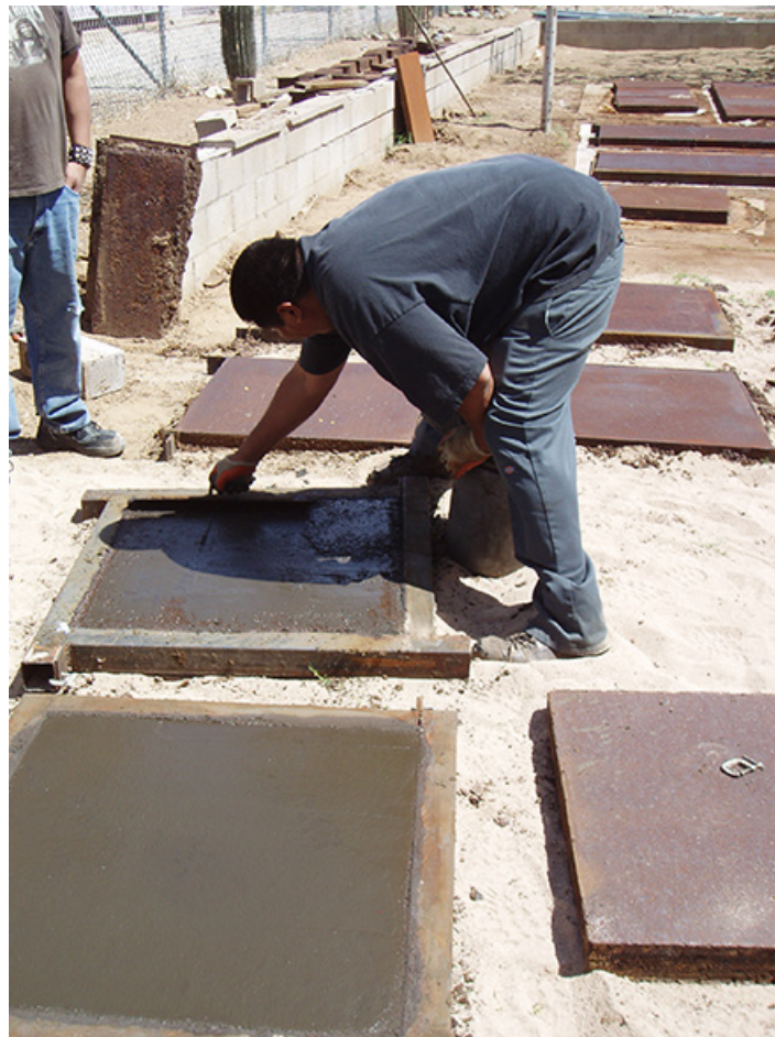
Tribal ecoAmbassador student intern setting building material into paver molds. Photo courtesy of TOCC.
