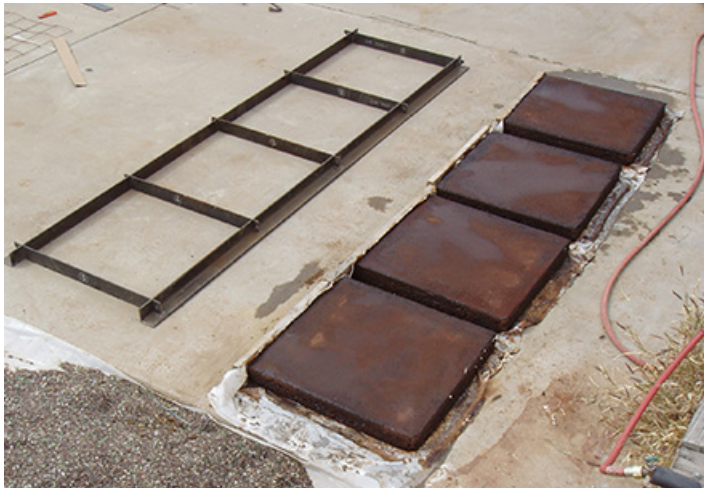
Large paver molds used to create pavers for TOCC Cultural Center patio. Photo courtesy of TOCC.
