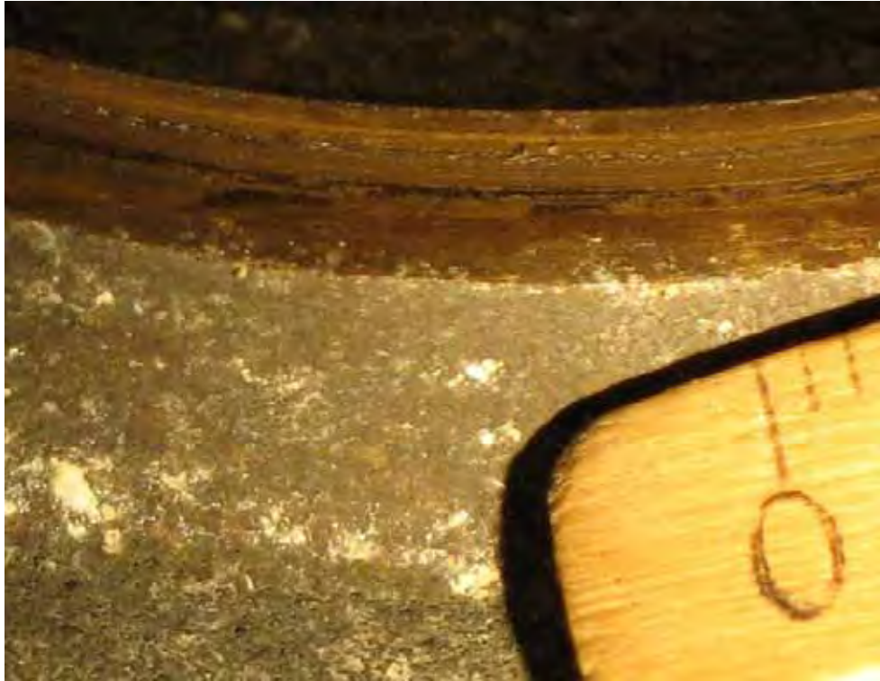
Figure C.83 Photograph of the bottom of meter 7.
