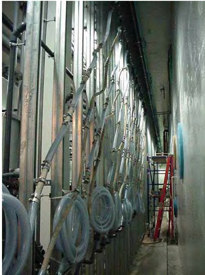
Figure C.87 Photograph of Washington Aqueduct Pipe Rack
