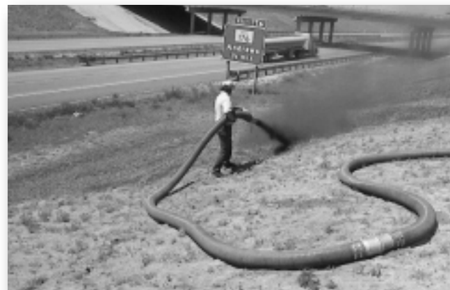
Figure 2 – Applying Compost
