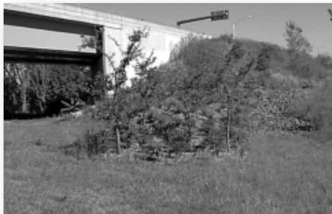
Figure 1 – I-91/Route 3 Interchange Plantings
