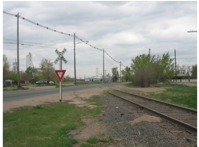
Site Identified for a new light rail station by the Commerce City Planning Department.
