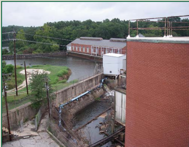
A view of Langdale Mill.
