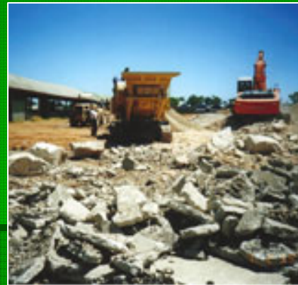
Crushed concrete as aggregate in new concrete
