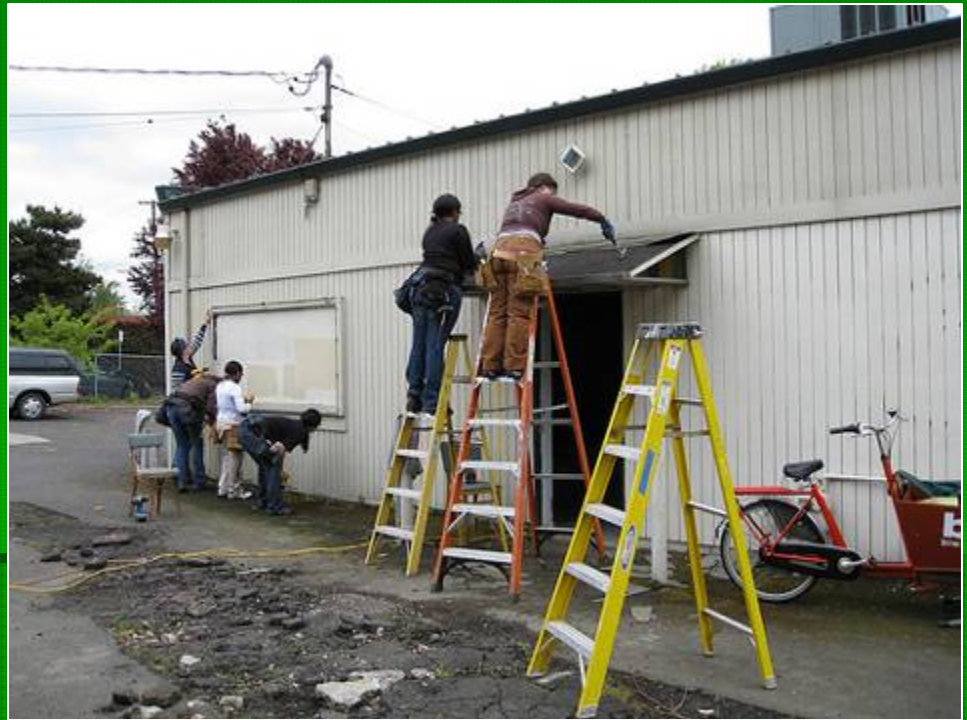
Students from Oregon Tradeswomen dismantle an awning and remove siding.
