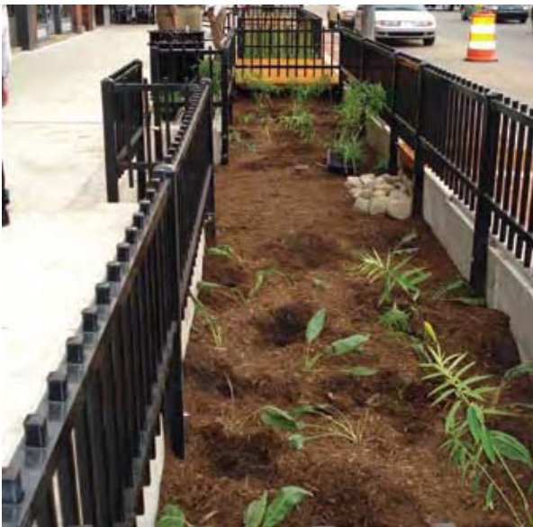
Street view of rain gardens in planter boxes in Lansing, MI. Source: Tetra Tech
