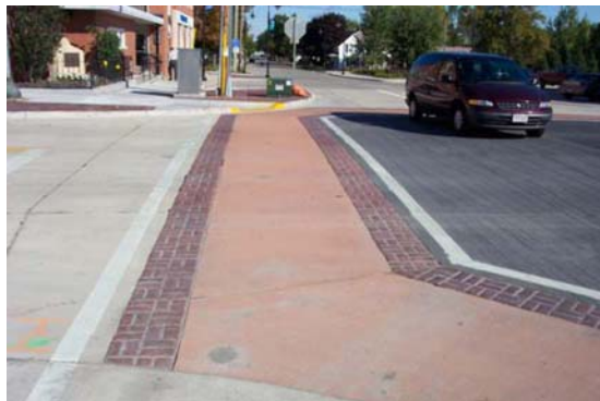
Colored Concrete crosswalk with brick paver edge
