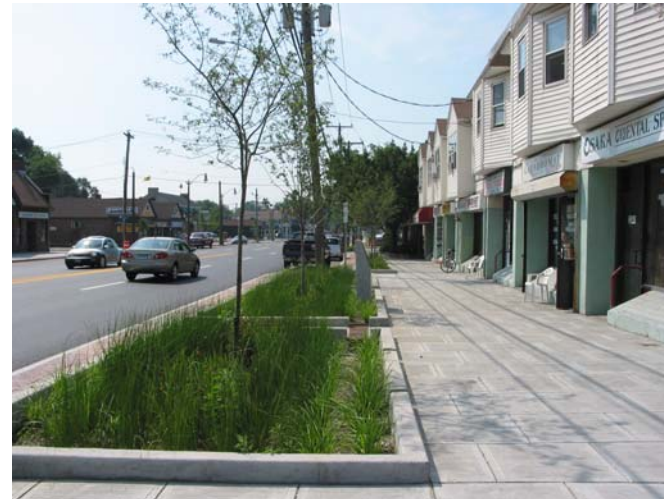
Sidewalk Stormwater Planter Photo Credit: www.tavelladesigngroup.com
