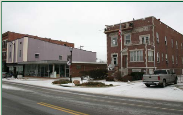
The historic Commercial Club Building in Springfield.
