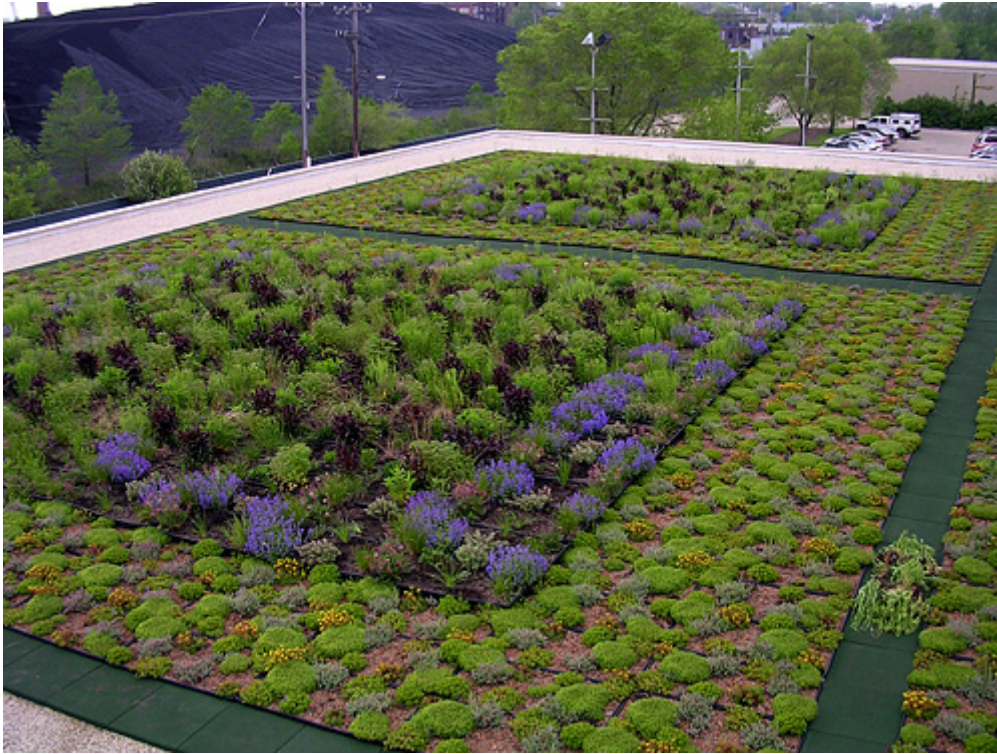
FIGURE 14: Example of modular drop-in-place system. 20
