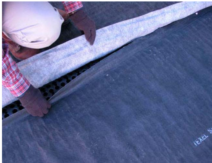
FIGURE 8: Filter fabric installed over plastic drainage layer. 14
