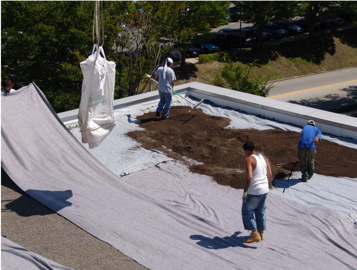
FIGURE 13: Built-in-place installation showing pea-gravel drainage, filter fabric, and growing medium. 19
