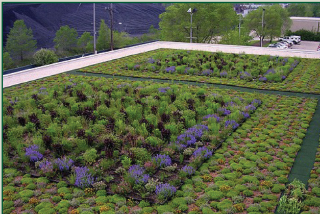
Example of a green roof. Photo source: Green Grid Roofs.
