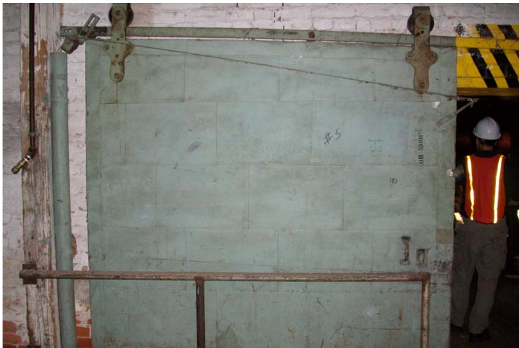
Photograph No. 5: Typical sliding track, wooden doors with pressed metal finish in Warehouse No. 5.
